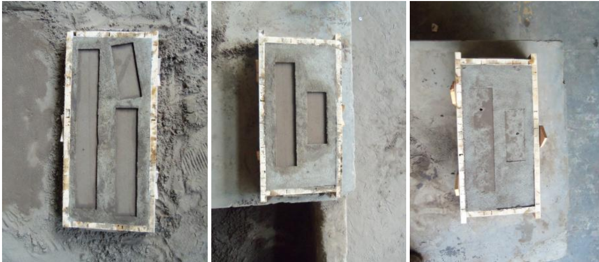
Figure 3.3: Preparation of mould for casting
