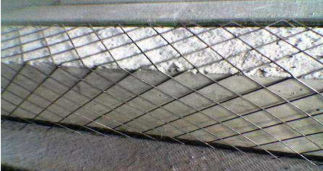
Figure 3.4 Orientation of Wiremesh at 45
