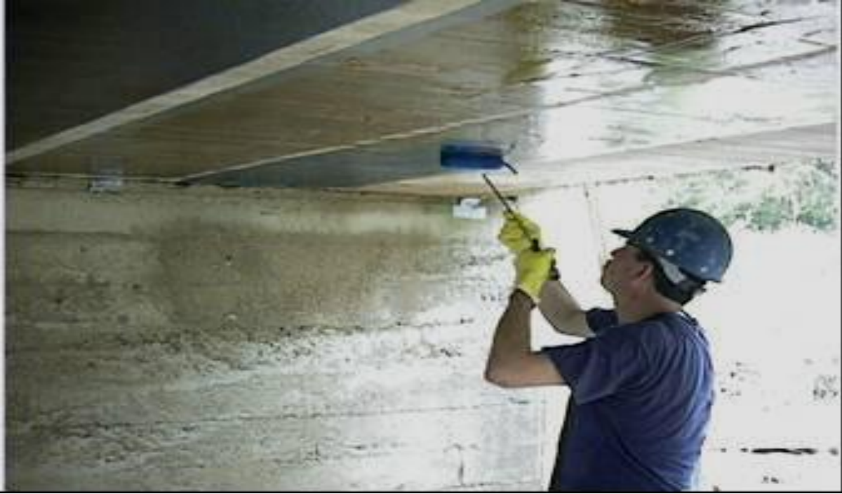
Figure 1.2 Fiber wrapping of the slab [15]
