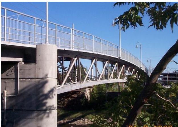
Fig.1.7 (a): Sherbrooke footbridge
