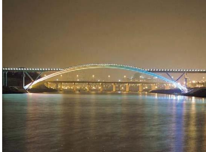
Fig 1.8 (a): General view of Seoul footbridge [Karmout, M.; (2009)]
