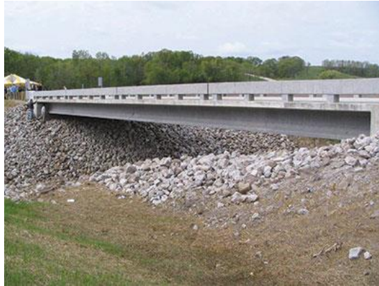
Fig: 1.6: UHPC Bridge at Wapello County
