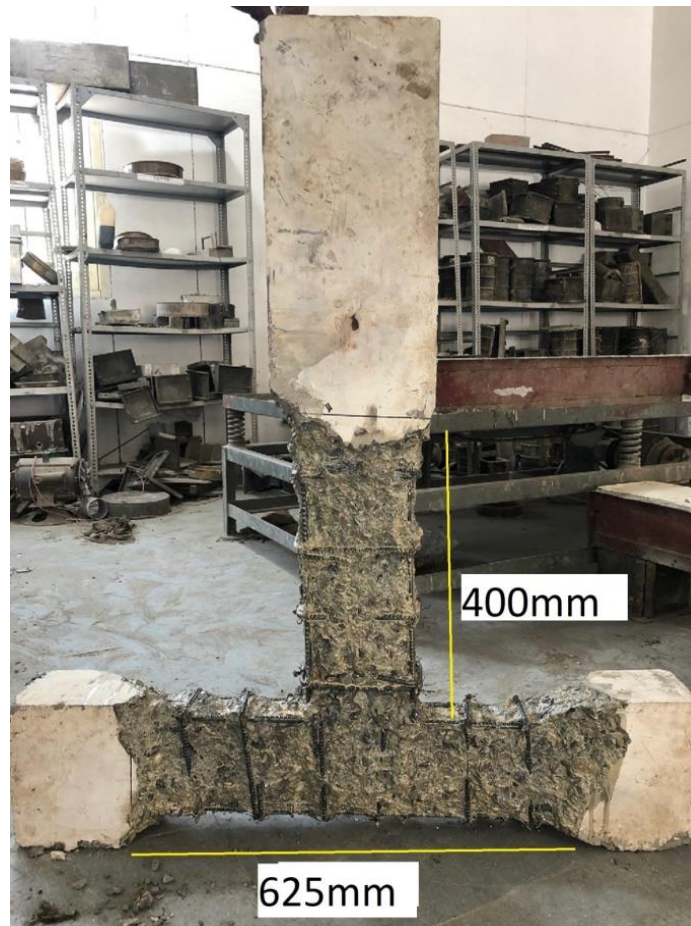
Figure 4.6 Geometric Dimension of The Chipped Area to Retrofit BJC Specimen
