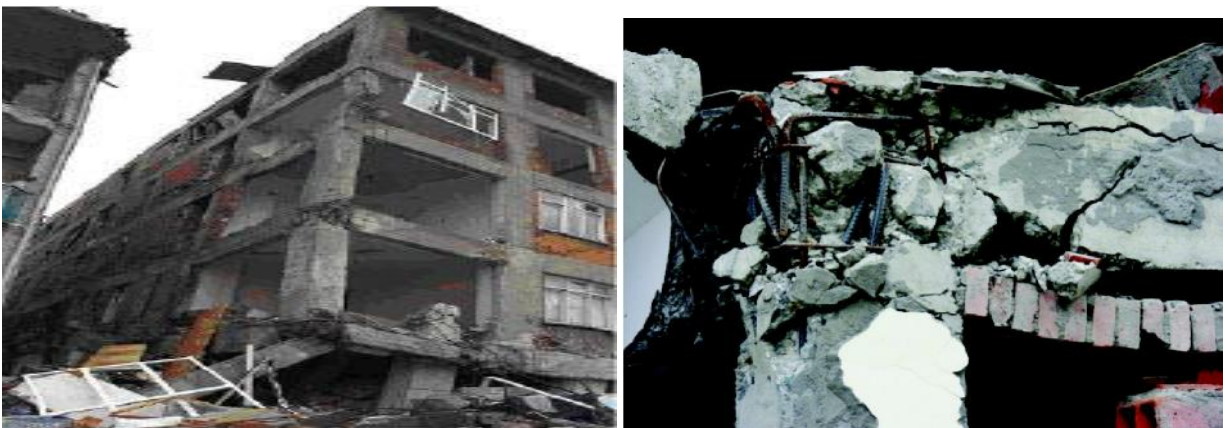
Figure 1.1 Exterior beam column joint failure in earthquake in Turkey1999 ( www.britannica.com )
