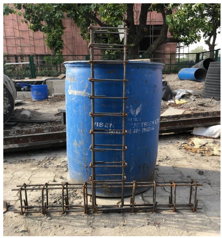
Figure 4.2 Reinforcement Detailing of Steel for T Beam
