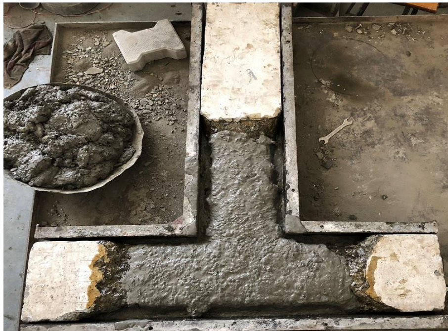
Figure 4.8 ECC Poured in Chipped Specimen Surface Placed in Form Work
