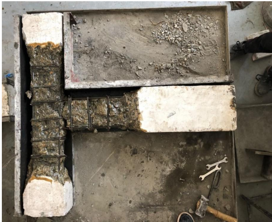
Figure 4.7 Nito Bond Layering on The Beam Column Chipped Surface Joint
