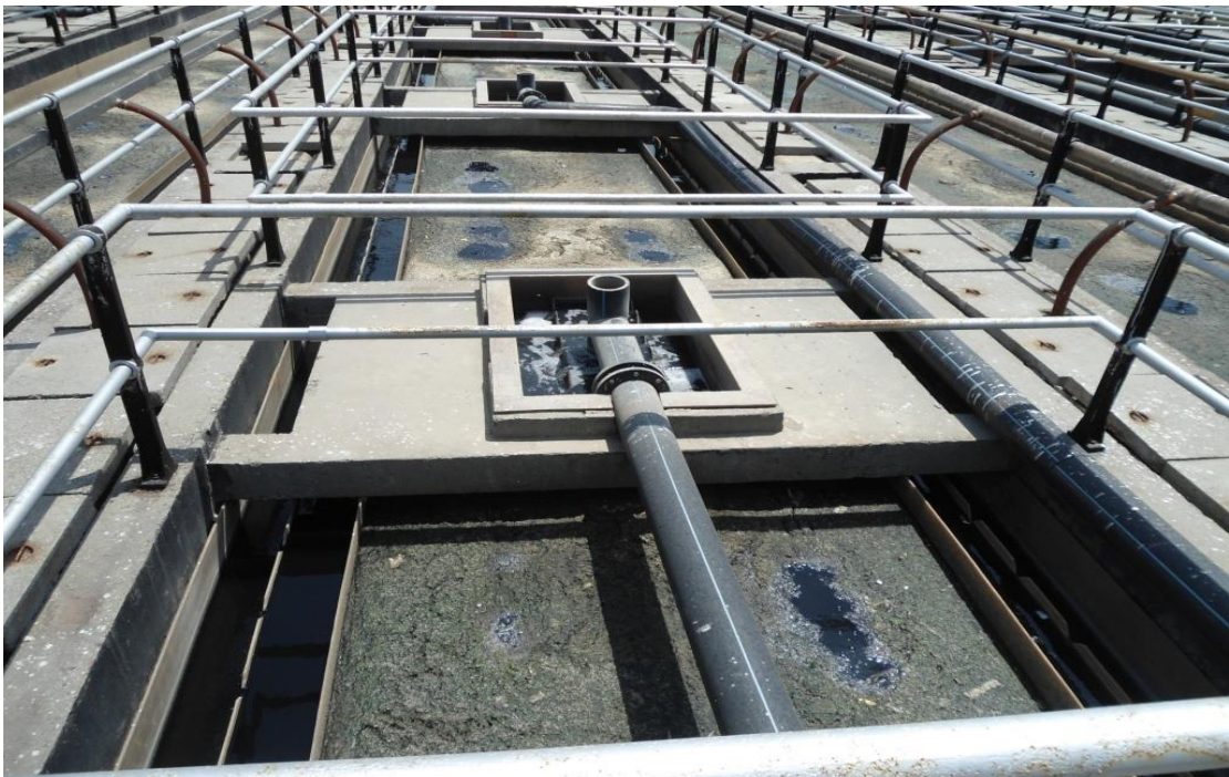
Figure 4.7: UASB reactors
