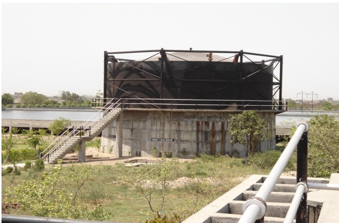
Figure 4.10: Biogas holder
