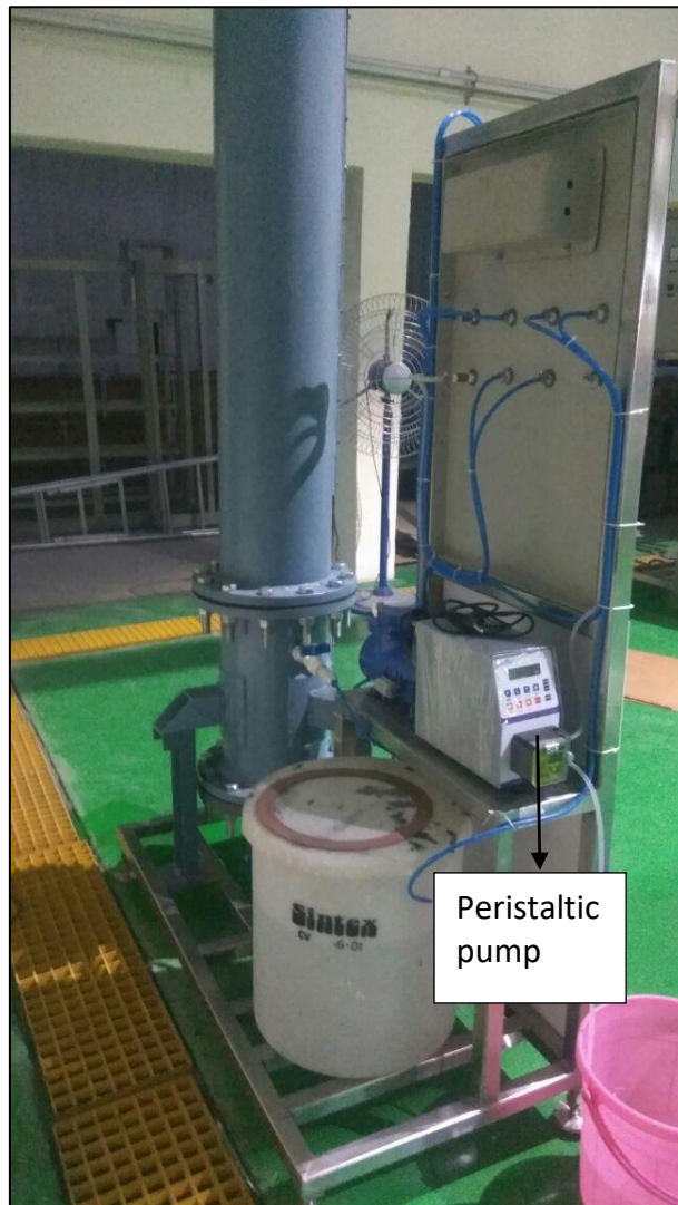
Figure 20 Erected biological aerating tower
