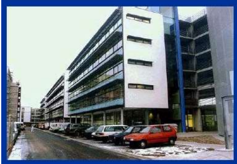
Figure 1.6 Vilbeler Beg office building, Darmstadt, Germany[Marinkovic (2002)]
