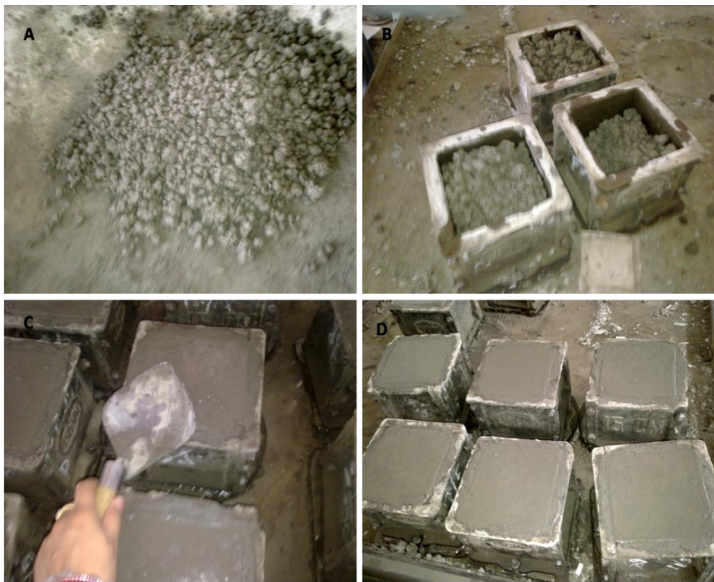
Fig 3.5: Casting of Concrete Cubes (M20)
