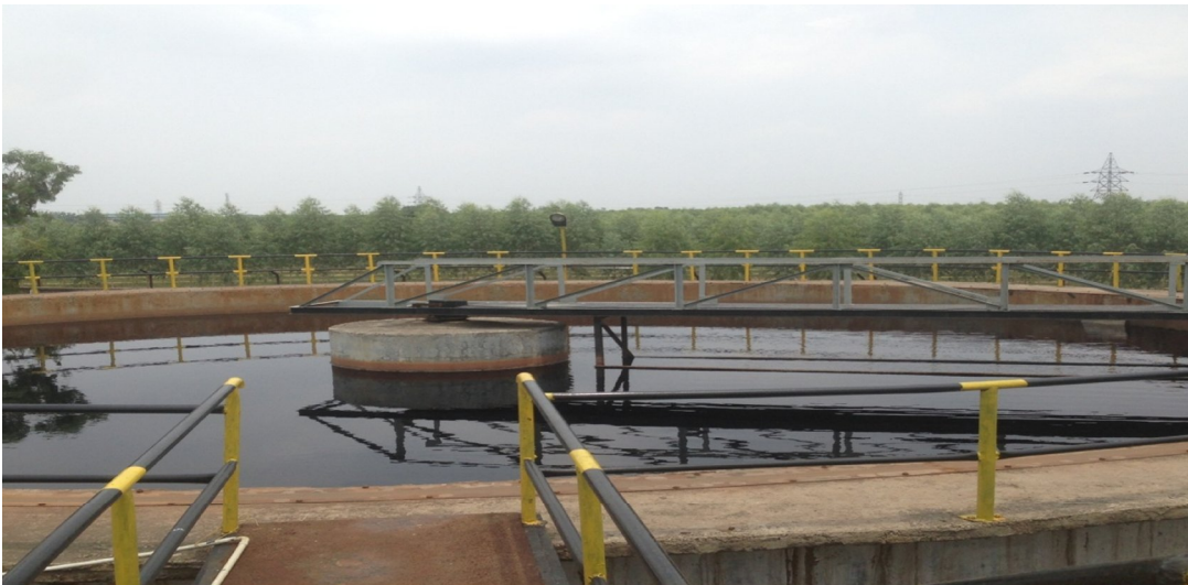
Fig 3.8 Secondary Clarifier
