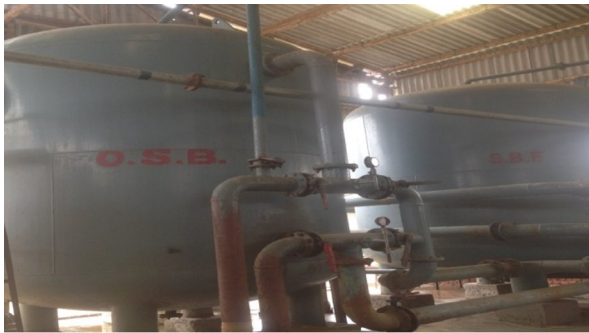
Fig 3.10 Filtration Unit
