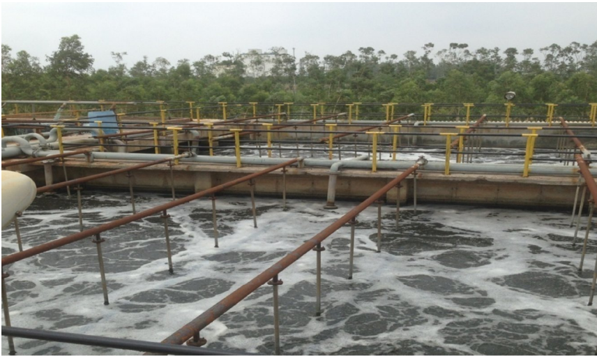
Fig 3.7 Aeration Tank
