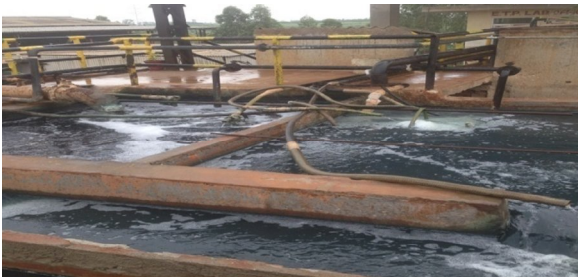
Fig 3.5 Flash mixing tank
