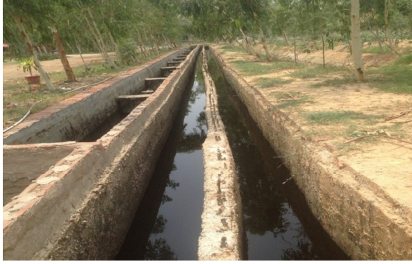
Fig. 3.1 Effluent receiving chamber
