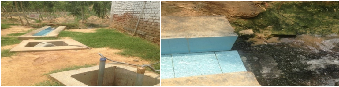
Fig 3.12 Reject water discharge in plantation area
