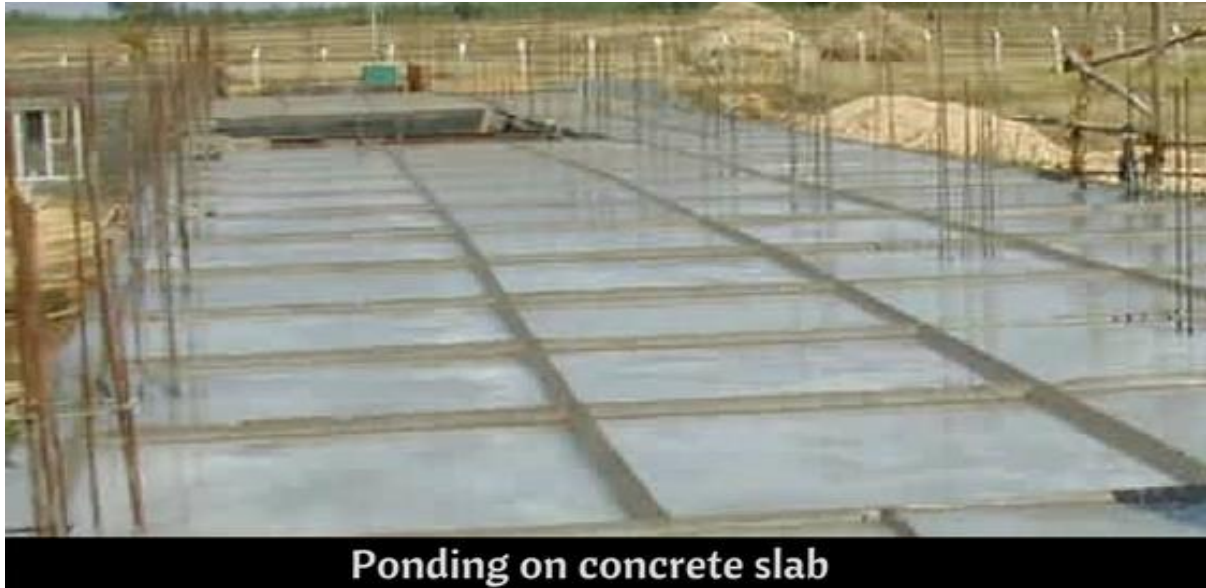
Figure 1.3: Curing of the concrete slab by ponding method
