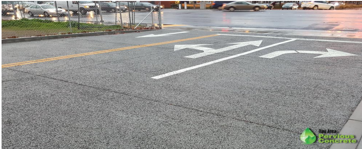
Figure 1.7: Pervious concrete pavement
