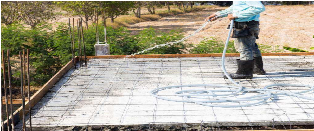
Figure 1.2: Water curing by sprinkling method
