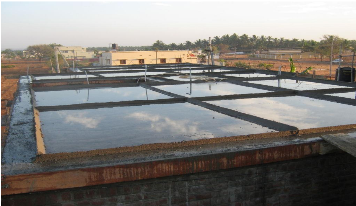
Figure 1.1: Curing of concrete
