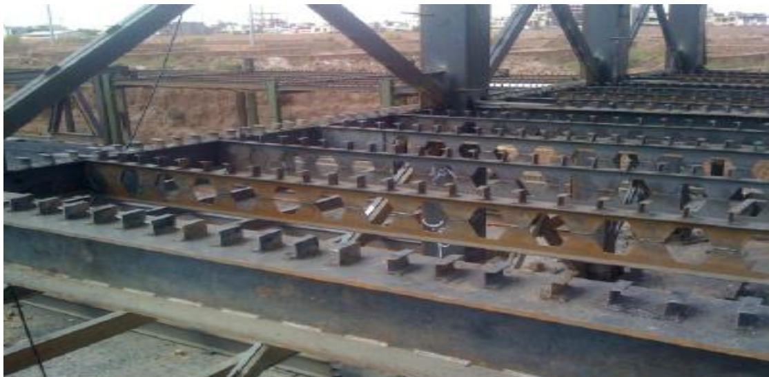
Figure 1- 2 Application of shear connector [32]
