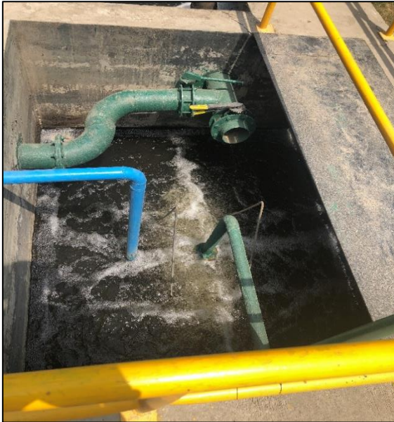
Figure 3-20 Top view of MBR Tank
