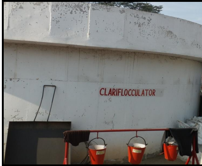
Figure 3-6 Side view of clariflocculator
