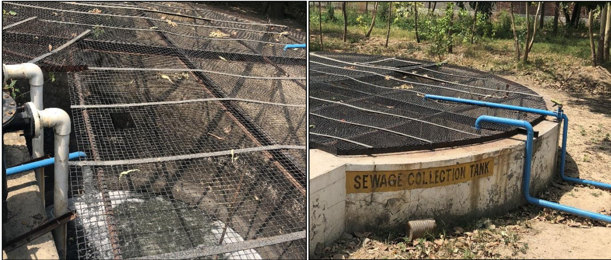
Figure 3-13 Sewage collection chamber
