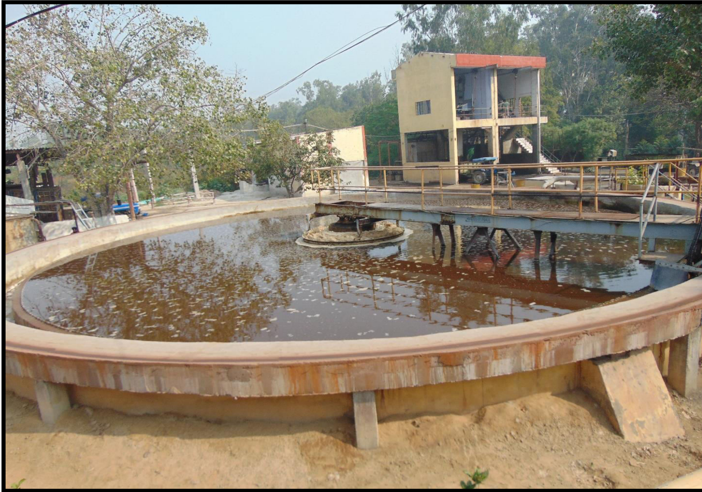
Figure 3.5 Industrial scale secondary clarifier
