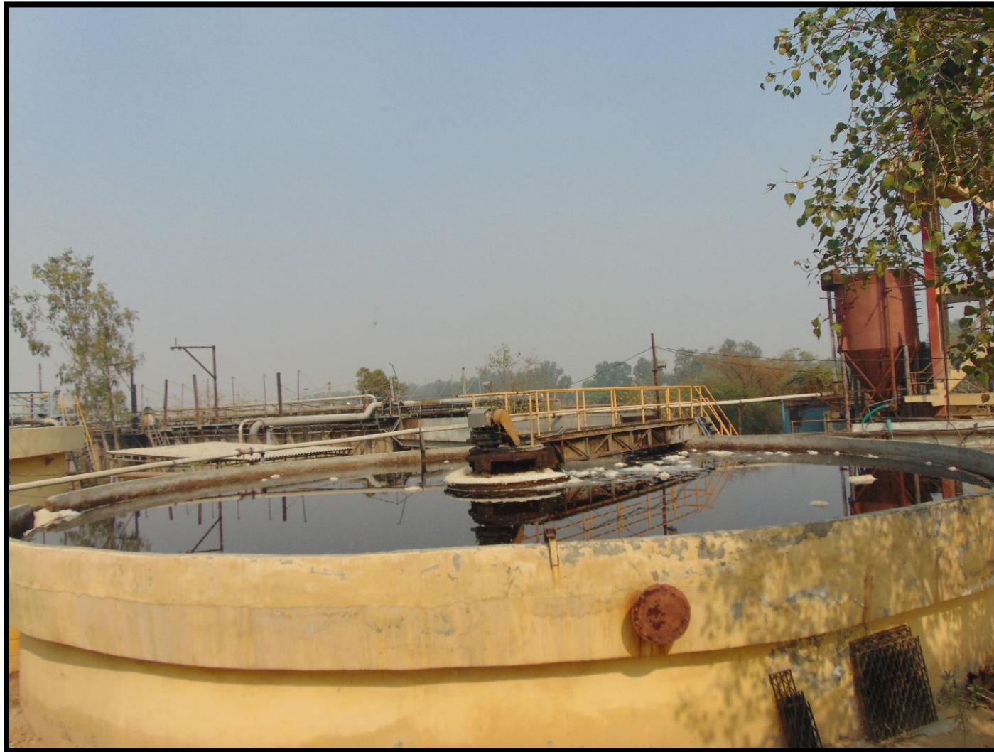
Figure 3.3 Industrial scale secondary clarifier-1
