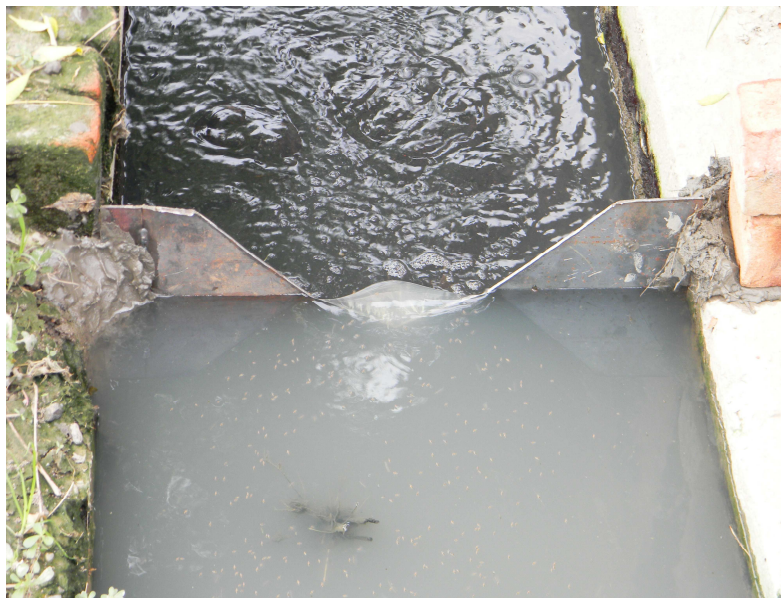
Figure 3.1: V-notch installed at Masitan village
