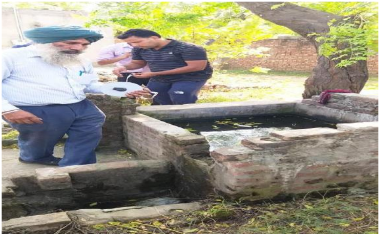
Figure 4.4 VALUATION of structure 1d
