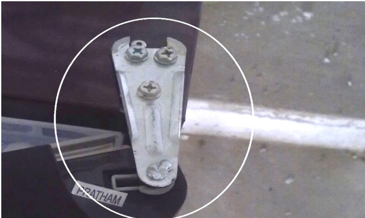
Figure 4.31: Existing door hinge
