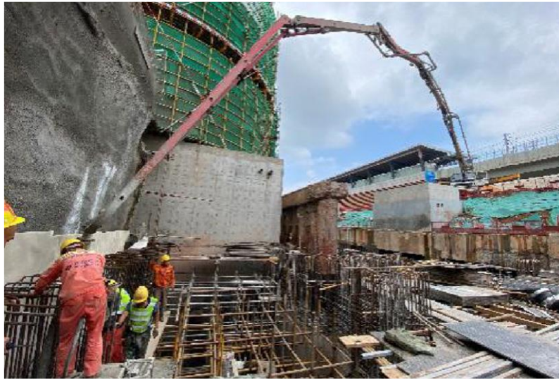
Figure 2.4: Pouring process of microbial self-healing concrete (Qian et al. 2021)
