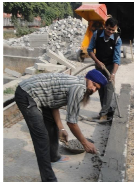
Plate 4.3: Concreting the RCC Beam Specimen (a) The Concrete Pan Mixer used for Preparing Concrete Mix; (b) Pouring and Vibrating the Concrete
