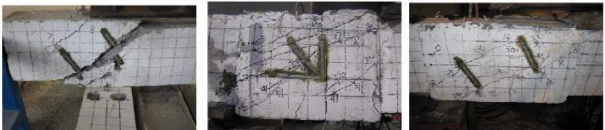
Plate 2.5: Cracking Pattern of BS-1, BS-2 and BS-3 Beams
