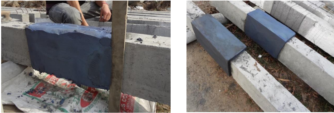
Plate 4.13: Application of PMF Jacketing on the Soffit and Side Faces of the Beams (by turning the beams upside down)
