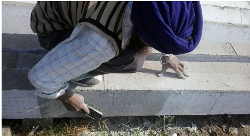
Plate 4.12: Preparation of Surface before Strengthening
