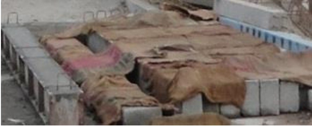
Plate 4.4: Curing of RCC Beam Samples
