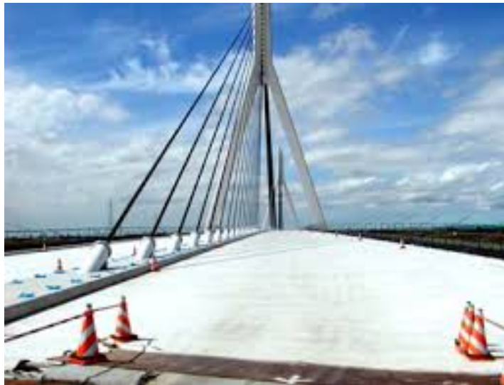
Figure 1.3: The Mihara bridge Japan uses a steel/SHCC composite deck (Victor 2006)
