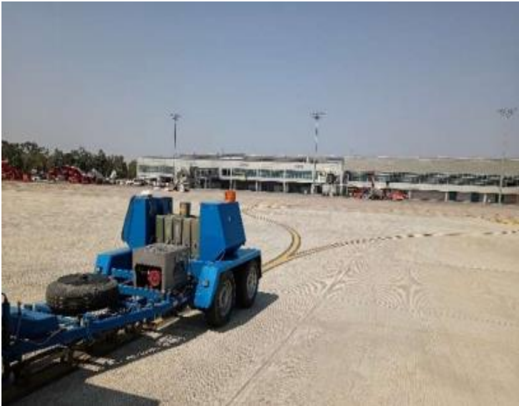
Fig 5. 6 Another view of Heavy deflectometer testing in progress on Stand 40 Rigid.
