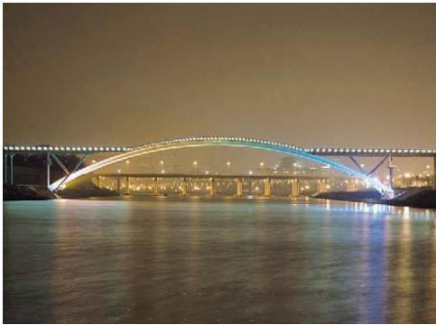
Fig 1.8 (a) General view of Seoul footbridge
