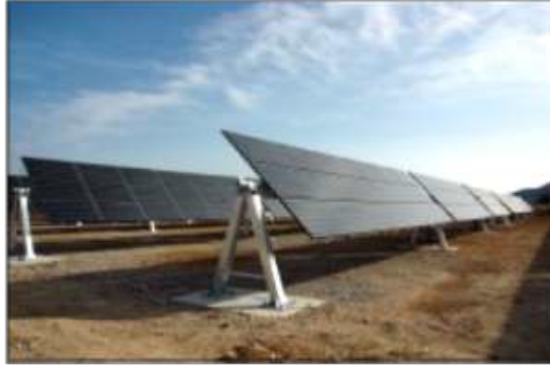
Figure 1.4: Single axis tracker [5]
