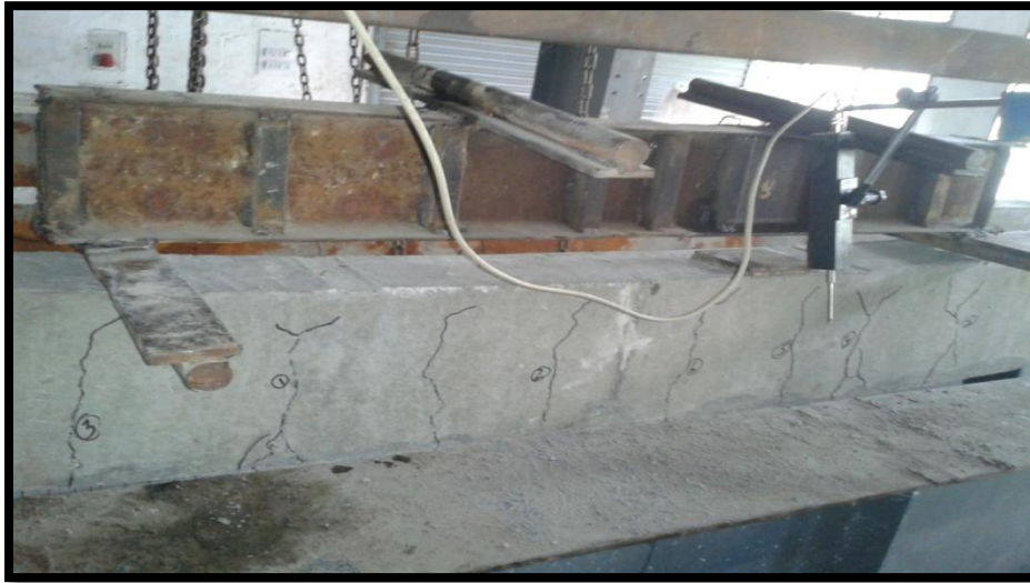
Fig: 5.15 Flexure Cracks on side face of C-0 beam
