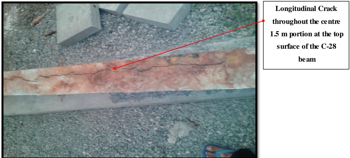
Fig: 5.1 (b) Longitudinal Crack on top surface of C-28 beam
