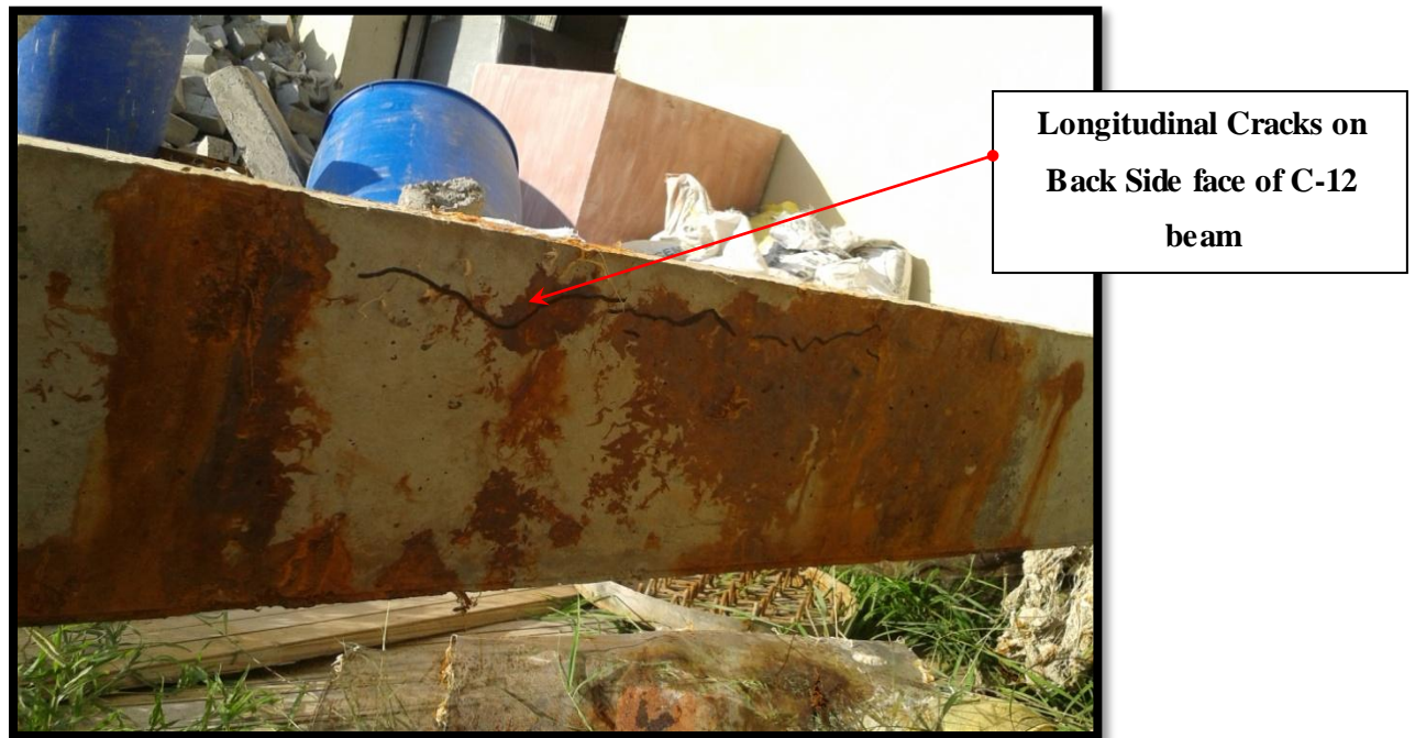
Fig: 5.10 Back Side Face of C-12 beam
