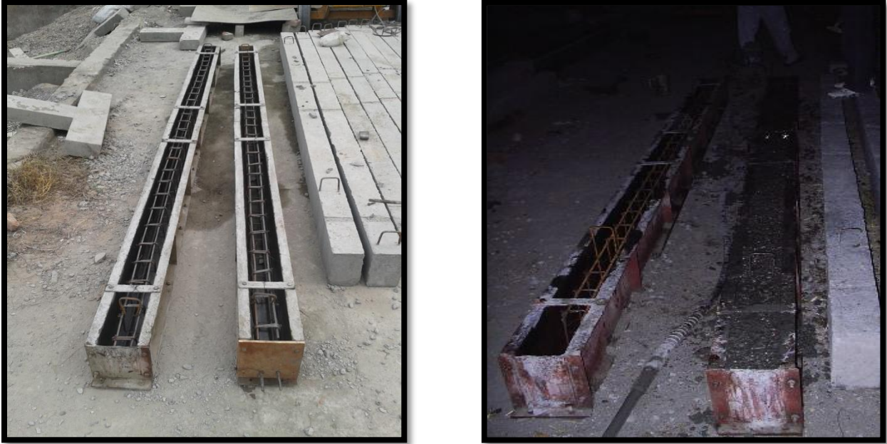
Fig. 4.2 Beams Before and After Casting
