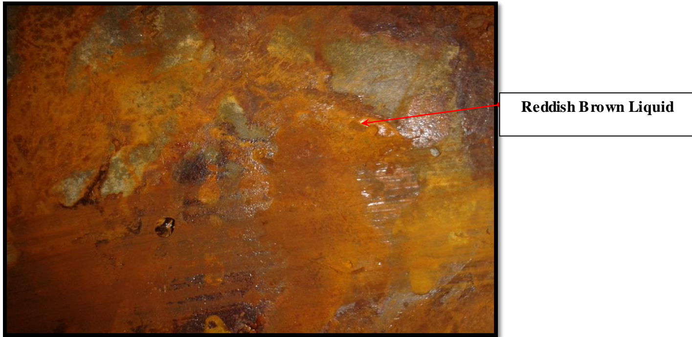
Fig: 5.14 back Side face of C-18 Beam
