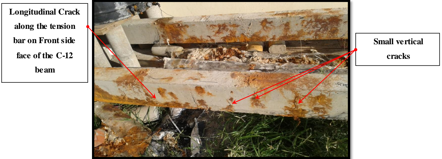
Fig: 5.9 Front Side Face of C-12 beam
