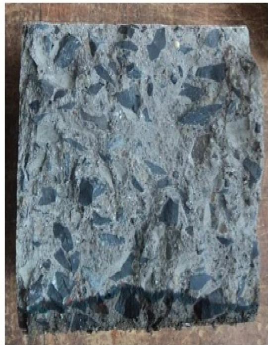
Figure 3.16 Water penetrated Sample
