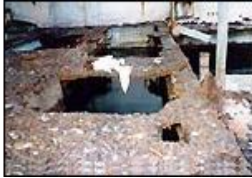
Fig. 1.6: Generalized Corrosion or Uniform Corrosion [4]
