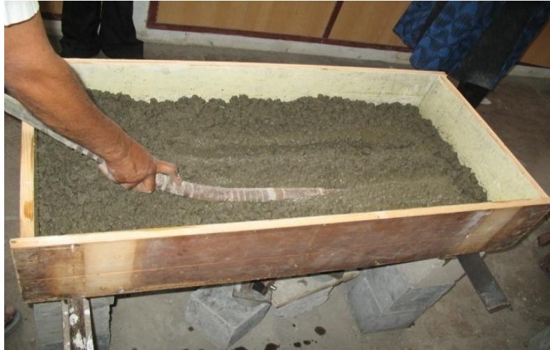
Fig.6.14. Use of needle vibrator
