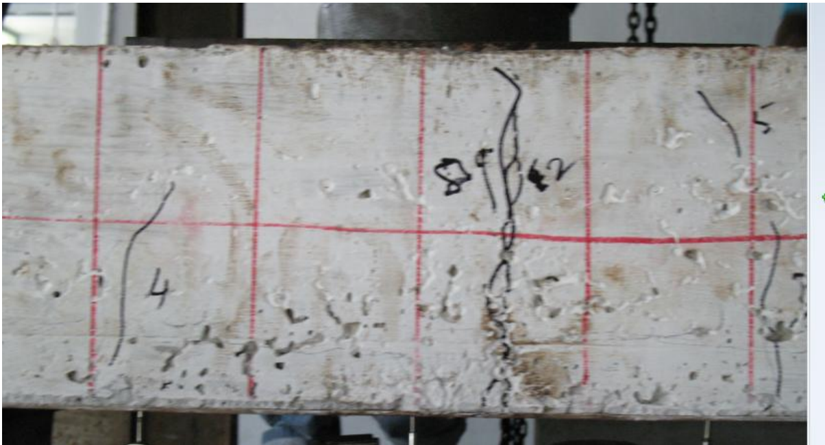
Fig.7.33 More cracks at load of 150 KN
