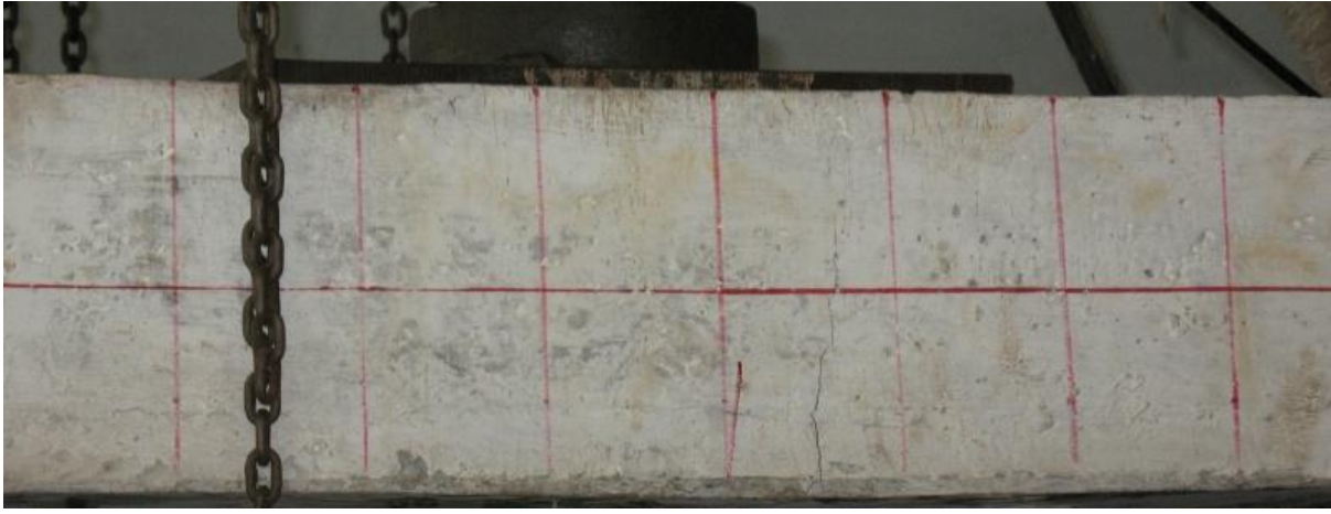
Fig.7.38b First crack in F21 slab
