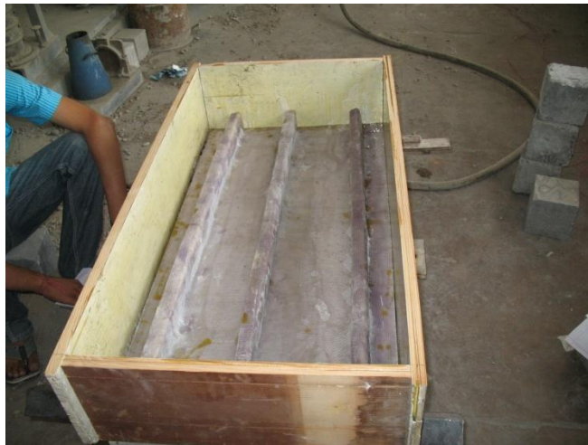
Fig.6.13. Side forms around the base form
