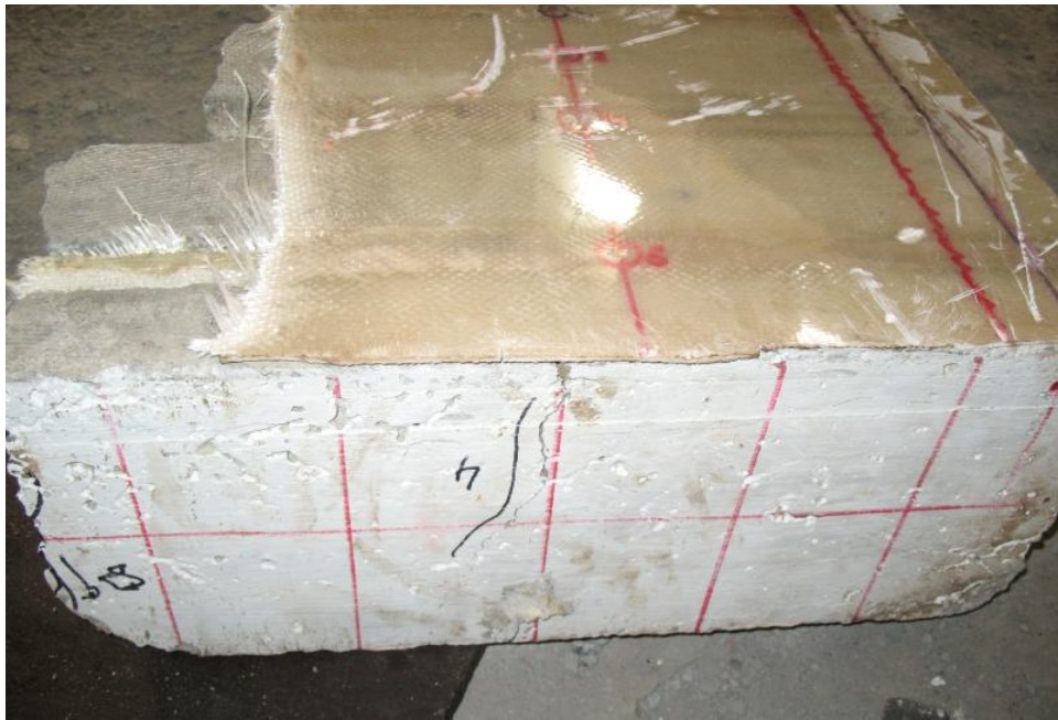
Fig 7.37 Delamination of channels
