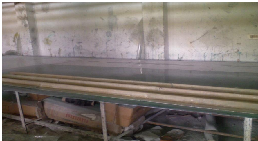
Fig.5.13. Three 1m span forms placed adjacent to each other before connection
