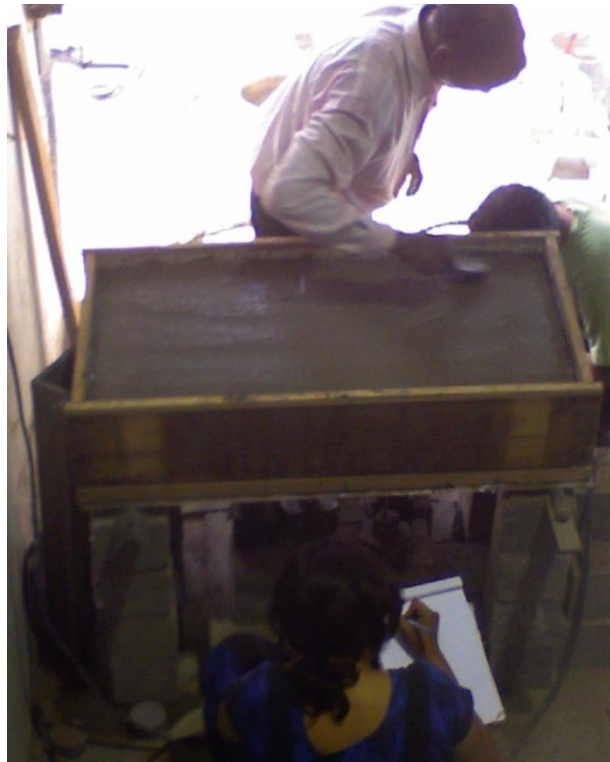
Fig.6.10. Slab casted on form F11
