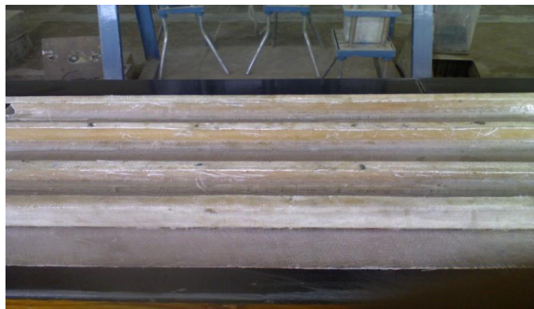
Fig.5.19. Four layer base form stiffened with channels
