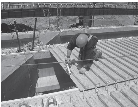
Fig.3.30. Installation of CDS deck panels
