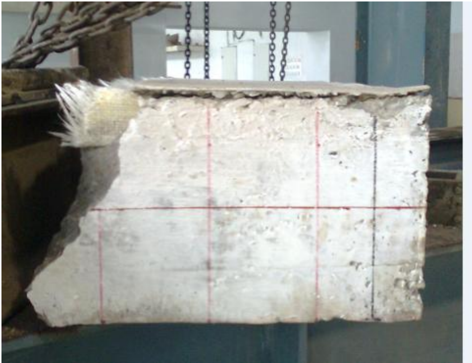
Fig.7.40 Delamination of form F21
