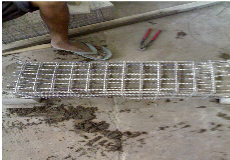
Plate -3. 4: Wrapping of wire mesh on beam
