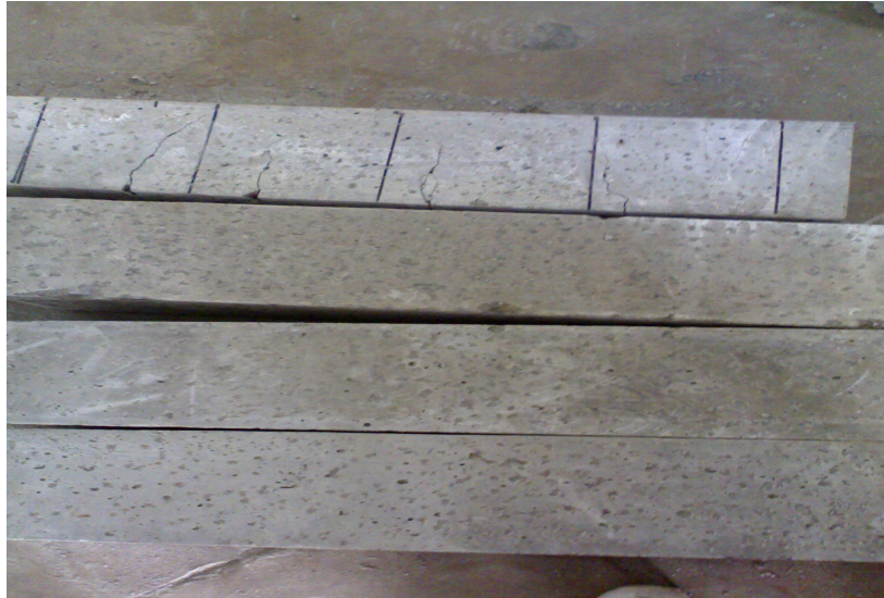
Plate – 3.3: Pitching of beams
