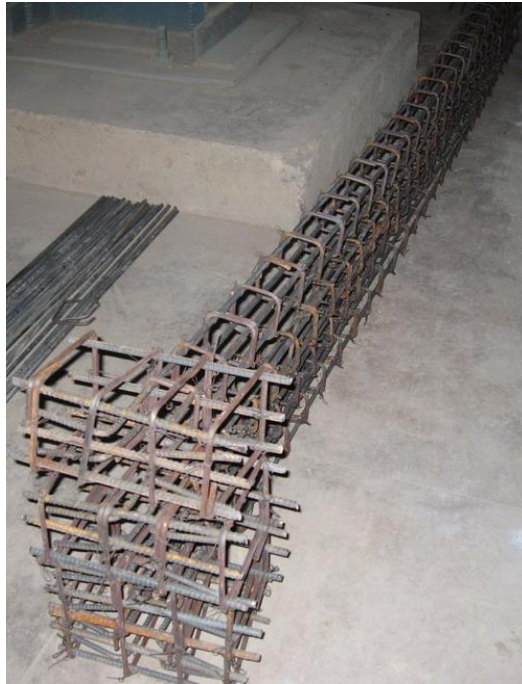
Figure 3.19 Column detail with stub of frame 1 and 2
