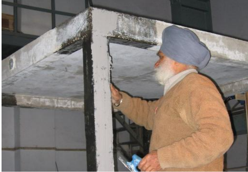
Figure 3.27 Applied MBrace Putty
