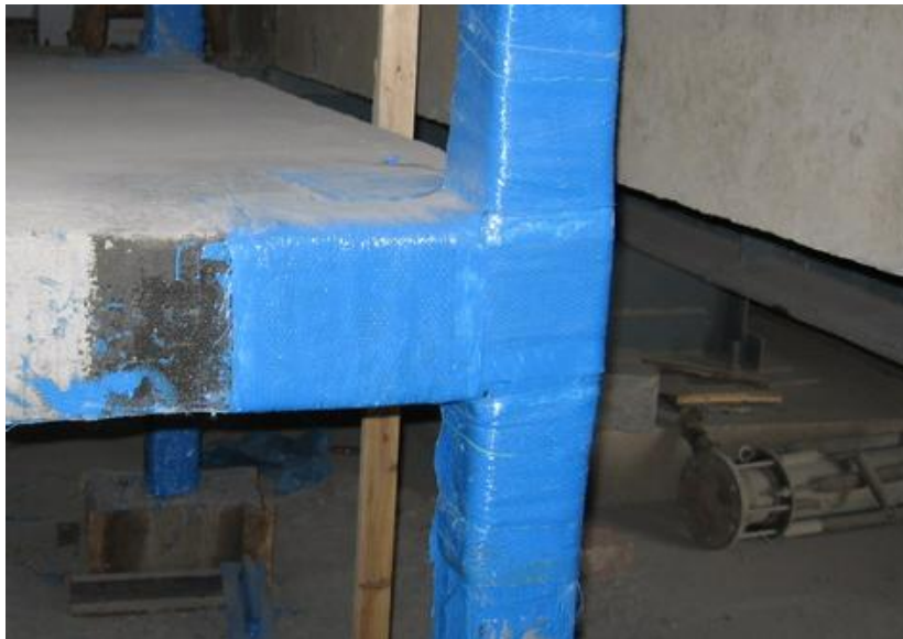
Figure 3.28 Applied MBrace Saturant with GFRP wrap
