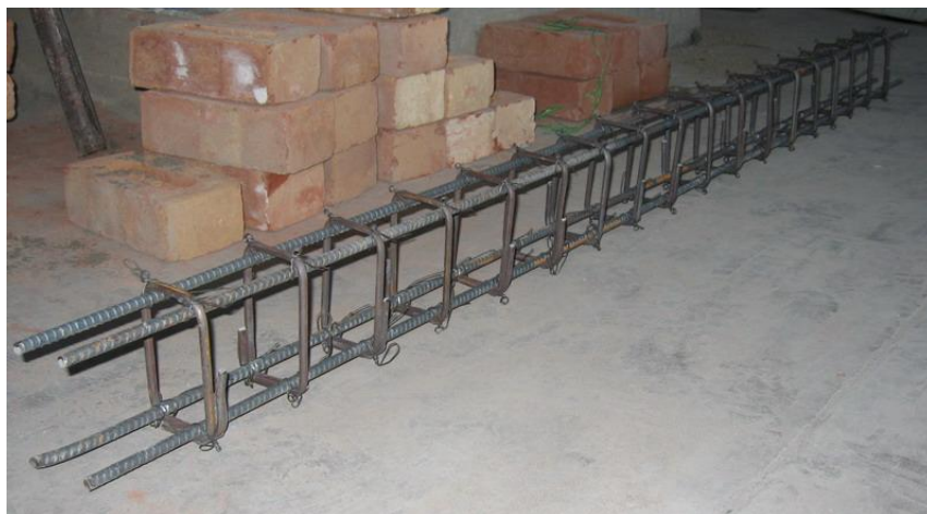
Figure 3.18 Beam detail of frame 1 and 2
