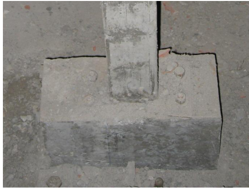
Figure 3.21 Foundation detail: column with stub
