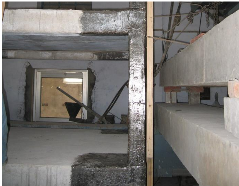
Figure 3.26 Applied MBrace Primer
