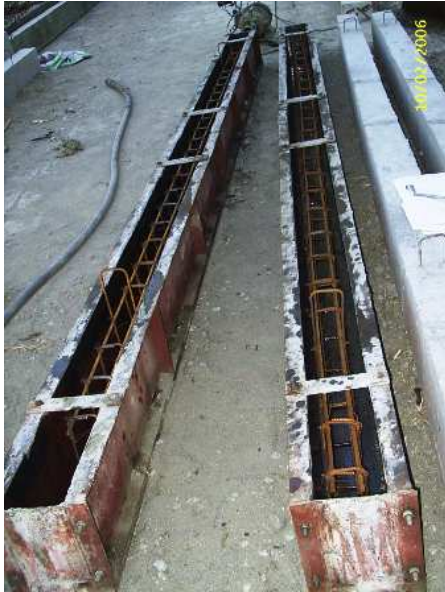
Plate-3.1: Beams Before and After Casting
