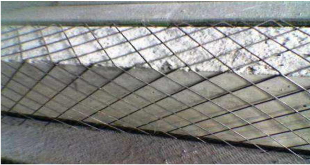
Plate 3.5: Beam with wire mesh at 45 degree
