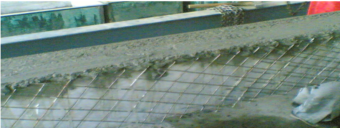
Plate 3.4: Beam with wire mesh at 60 degree
