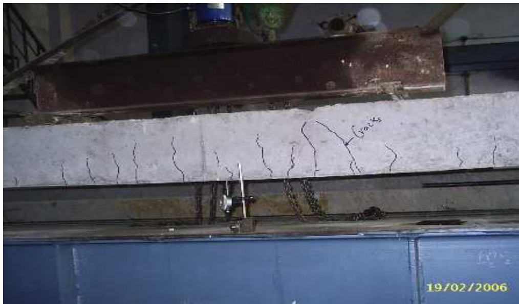
Plate-3.2: Failure of control beam
