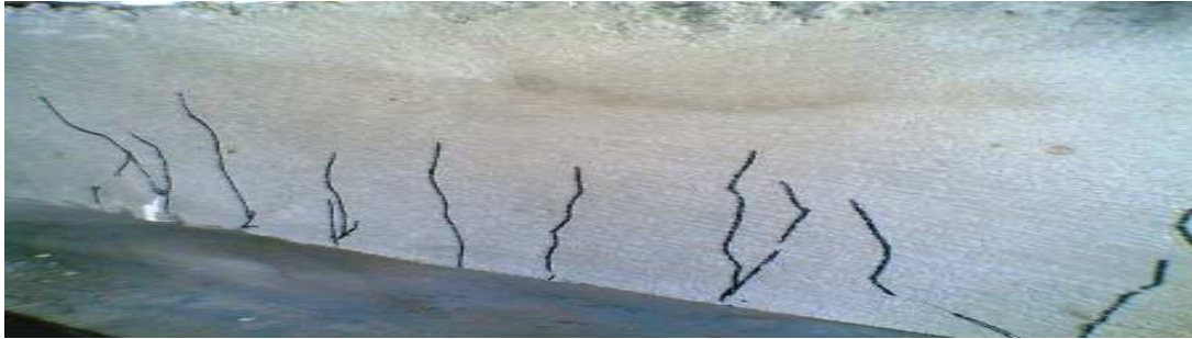
Plate 4.3: Crack Pattern of Retrofitted Beam with 60 Degree Wire Mesh
