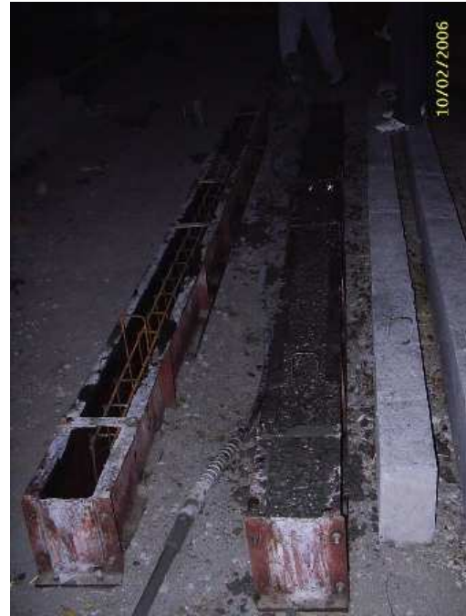
Plate-3.1: Beams Before and After Casting
