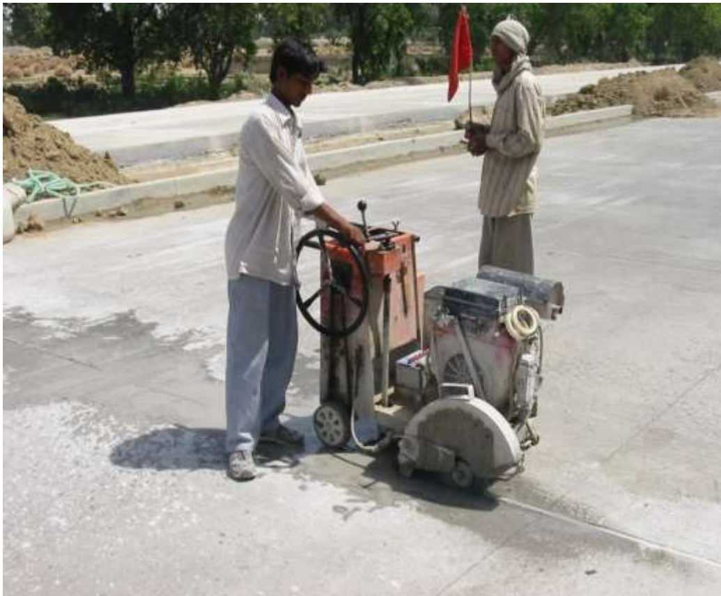
Fig. 1.4 Saw Cut in transverse direction
