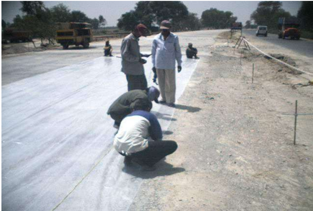
Fig. 1.2 Laying of separation membrane
