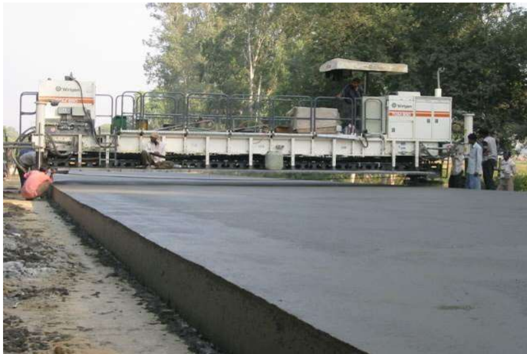
Fig. 1.9 Laying of Pavement Quality Concrete (PQC) with Slip Form Paver
