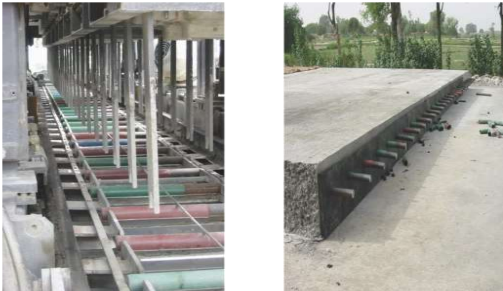
Fig. 1.7 Dowel bars in Pavement Quality Concrete (PQC)
