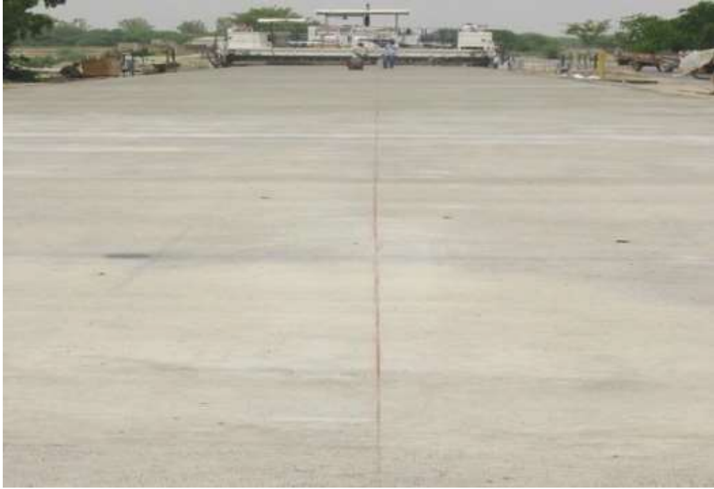
Fig. 1.3 Longitudinal joint in Pavement Quality Concrete (PQC)
