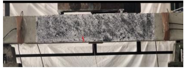
(a) Damage Level I
