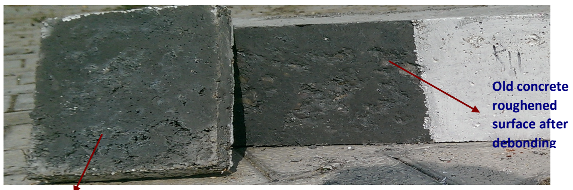
New UHPFRC layer debonding from the side face surface of old concrete surface
