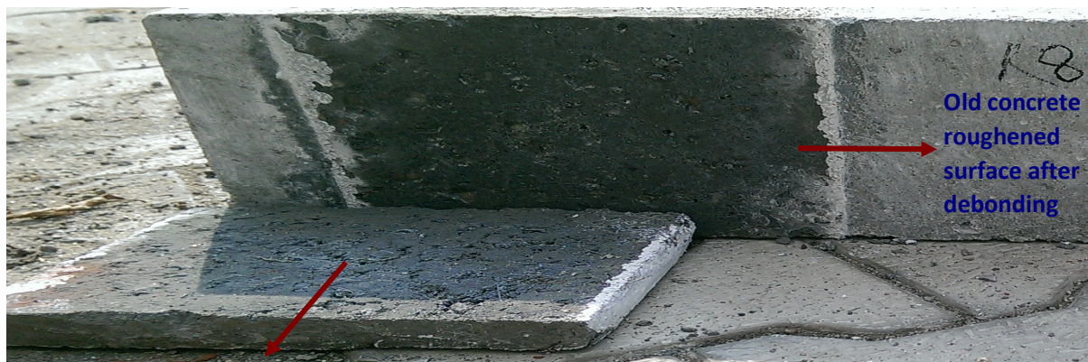
New UHPFRC layer debonding from the side face surface of old
