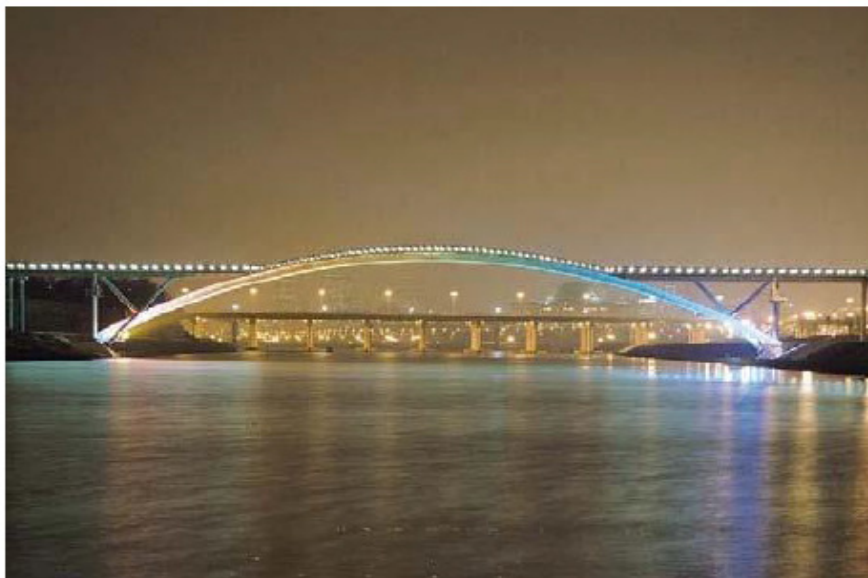
Fig 1.4 (a) General View of Seoul Footbridge [Karmout, M., (2009)]
