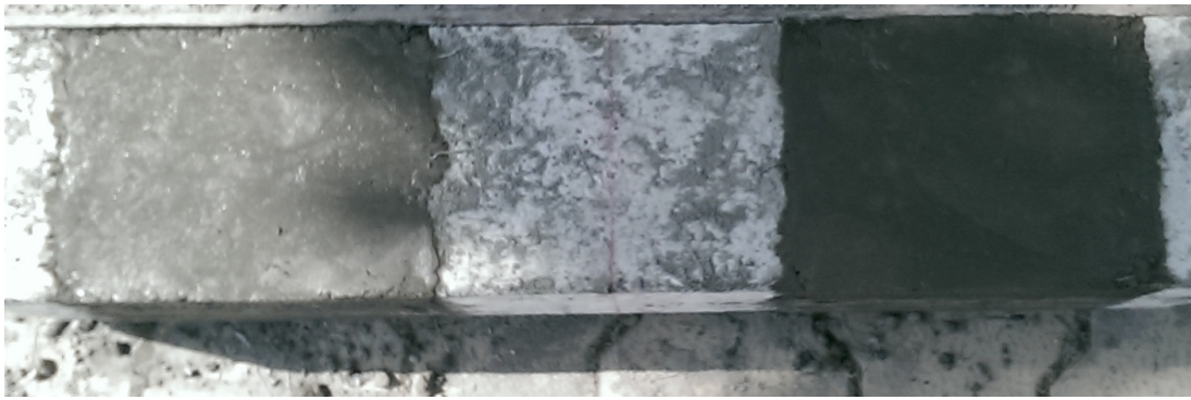
Fig. 3.11 Beam Retrofitted in U-Type Configuration (Stage 3)
