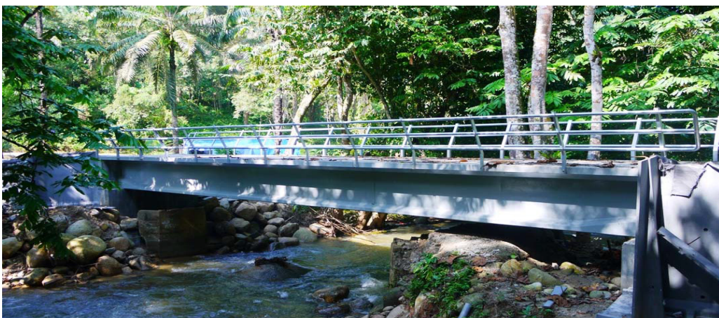
Figure 1.5 The New UHPFRC Bridge At Kampung Ulu Kampar, Gopeng, Perak.
