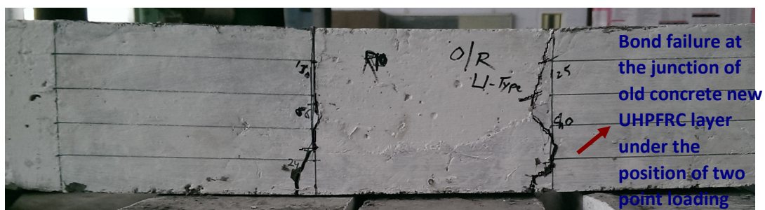
Fig. 4.18 Crack Pattern of Beam R10 at Failure
