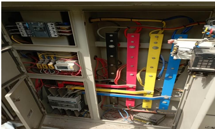
Fig 22 Installation of smart energy meters
