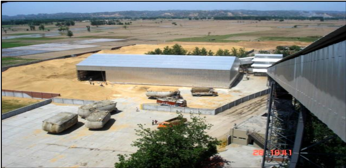
Fig. 3.3: Storage space and covered shed
