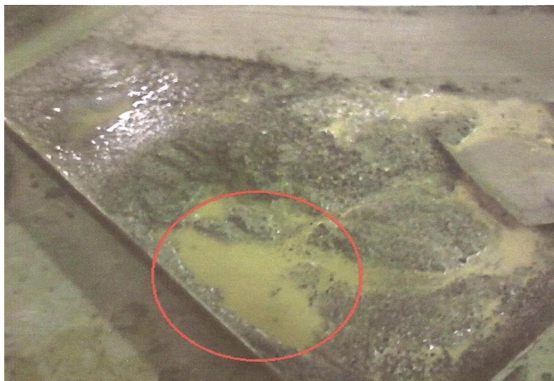
Plate 4.2 - Pools of water formed in mix G00
