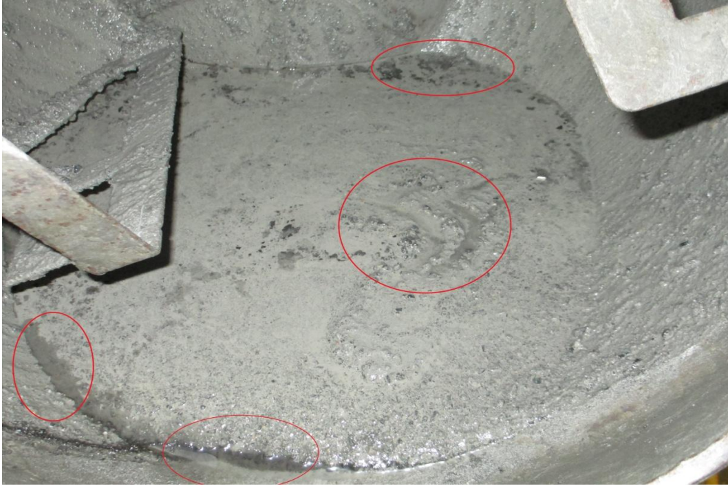
Plate 5.5 – Pools of water in the mixing drum (F4)
