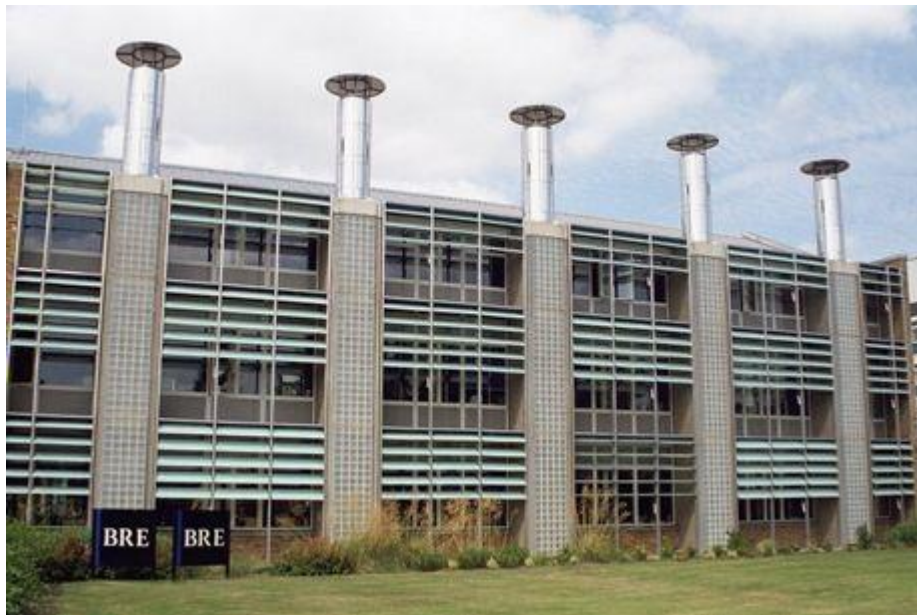
Fig 1.2: The BRE office building ( www.projects.bre.co.uk )
