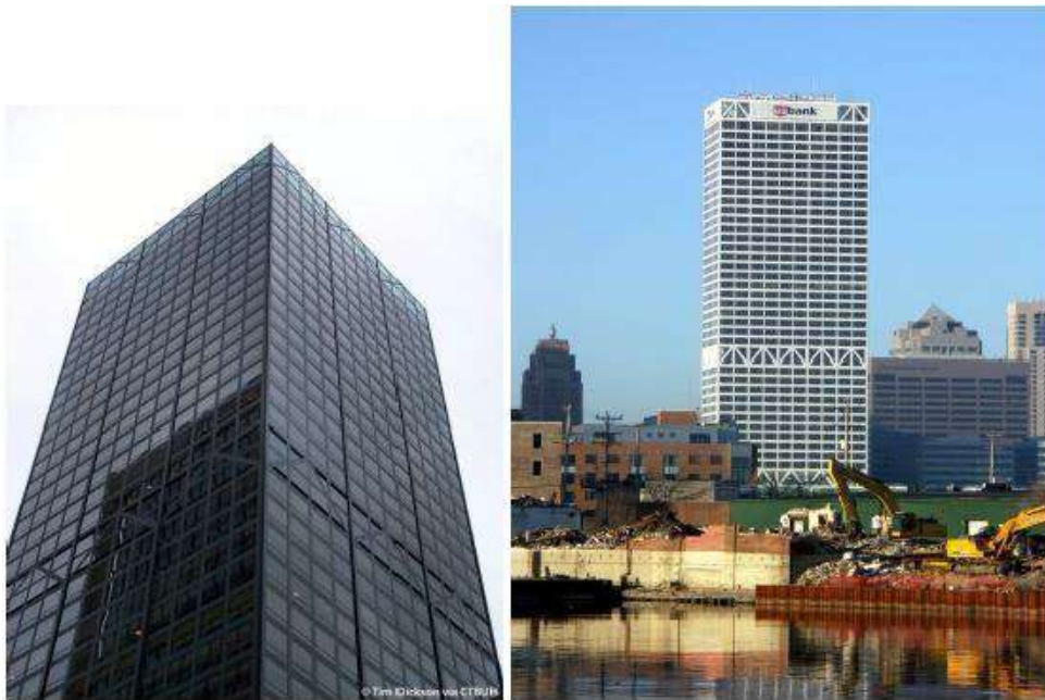
Figure 1. 9 Building with Outrigger System (Source: First Wisconsin Bank, designed by Fazlur Rahman Khan, Tokyo)
