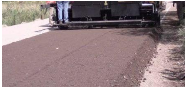
Figure 1-6 Providing base course
