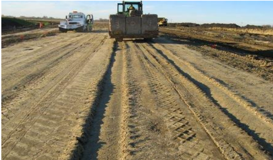
Figure 1-9 Preparing of sub-grade soil.
