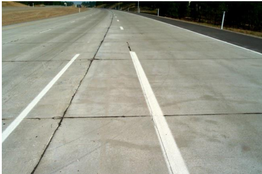
Figure 1-11 Pavement showing Longitudinal and Transverse joint
