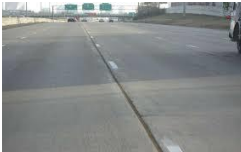
Figure 1-13 Concrete Pavement showing joint
