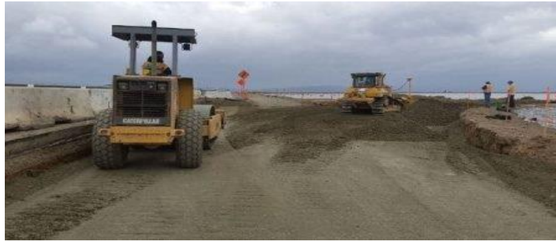
Figure 1-7 Laying of sub-base course.
