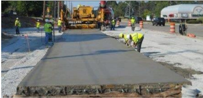
Figure 1-5 Concrete Slab Laying
