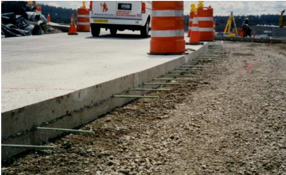
Figure 1-17 Tie Bars in Pavement
