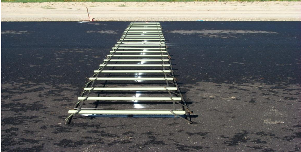
Figure 1-14 Arrangement of Dowel bars
