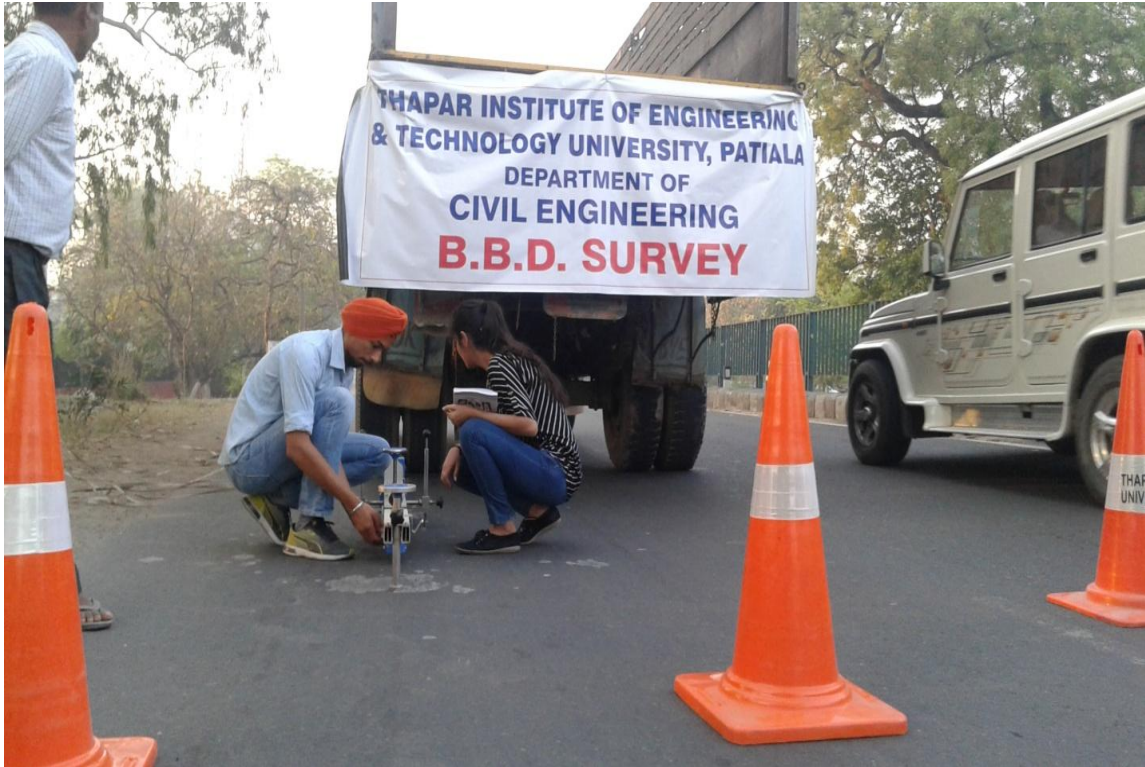
Figure 4.10: Benkelman Beam Deflection Test in Progress at Chainage 0.200 km, Section UR-02
