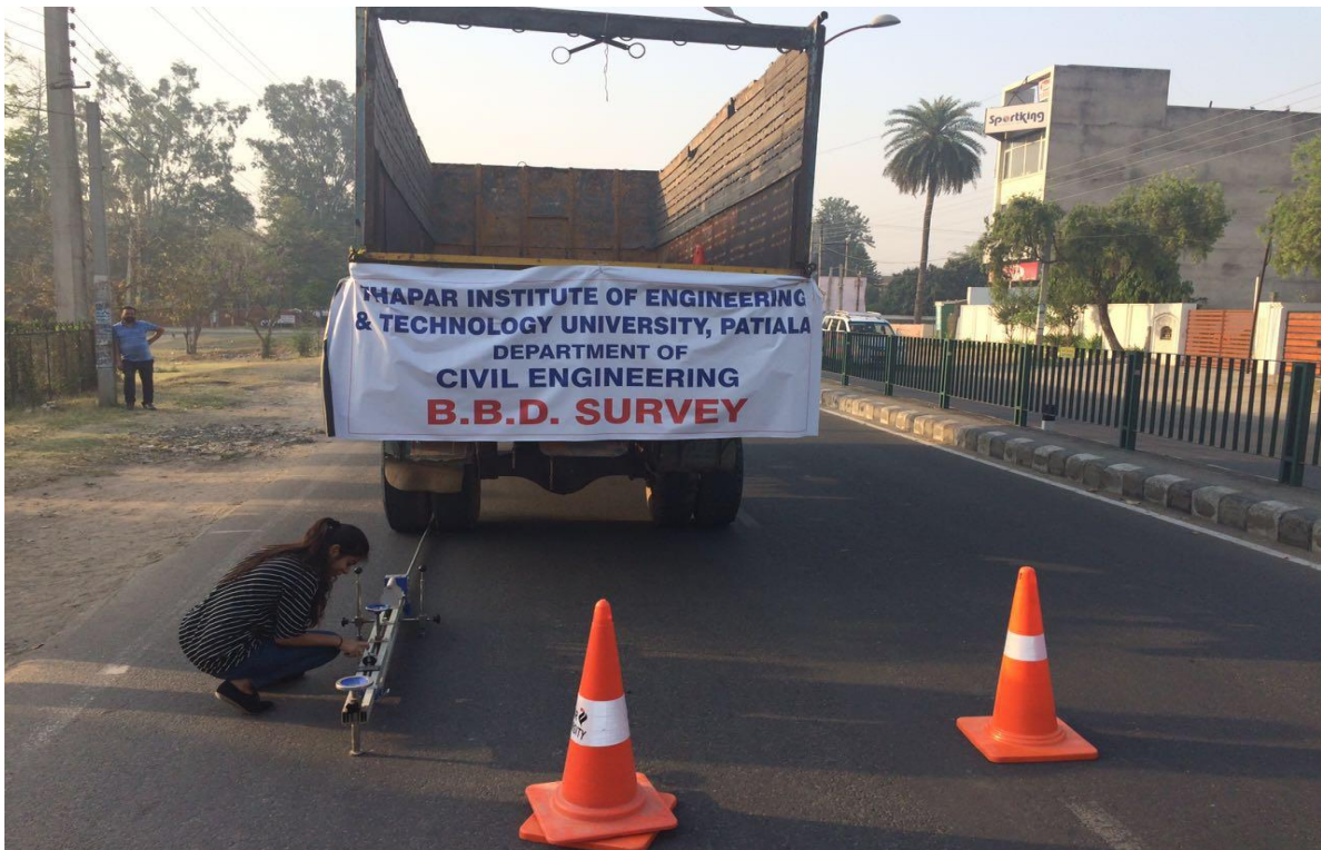
Figure 4.11: Benkelman Beam Deflection Test in Progress at Chainage 0.350 km, Section UR-02
