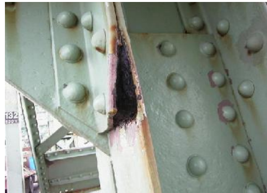
Figure 1.10 Crevice corrosion [18]
