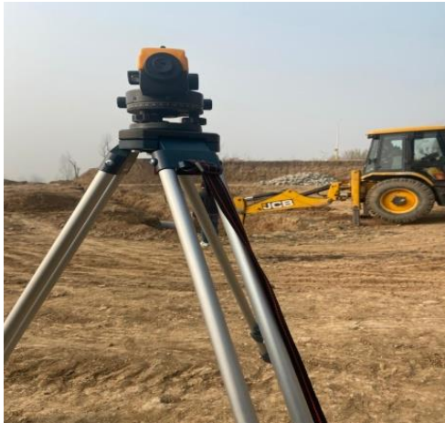
Figure 4.1: Leveling of site
