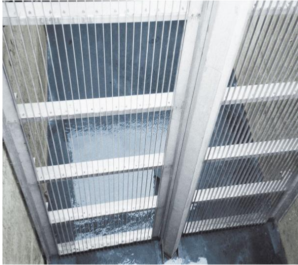
Figure 1.5: Coarse screen and Fine Screen
