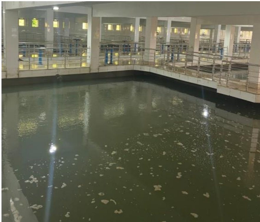
Figure 1.8: Sedimentation tank
