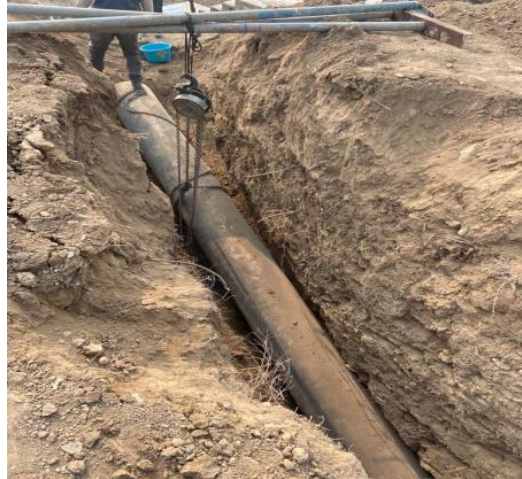
Figure 4.3: Laying of pipes
