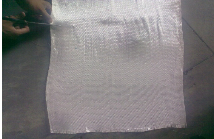
Fig. 4.9 Cutting of glass fibre sheet as per size
