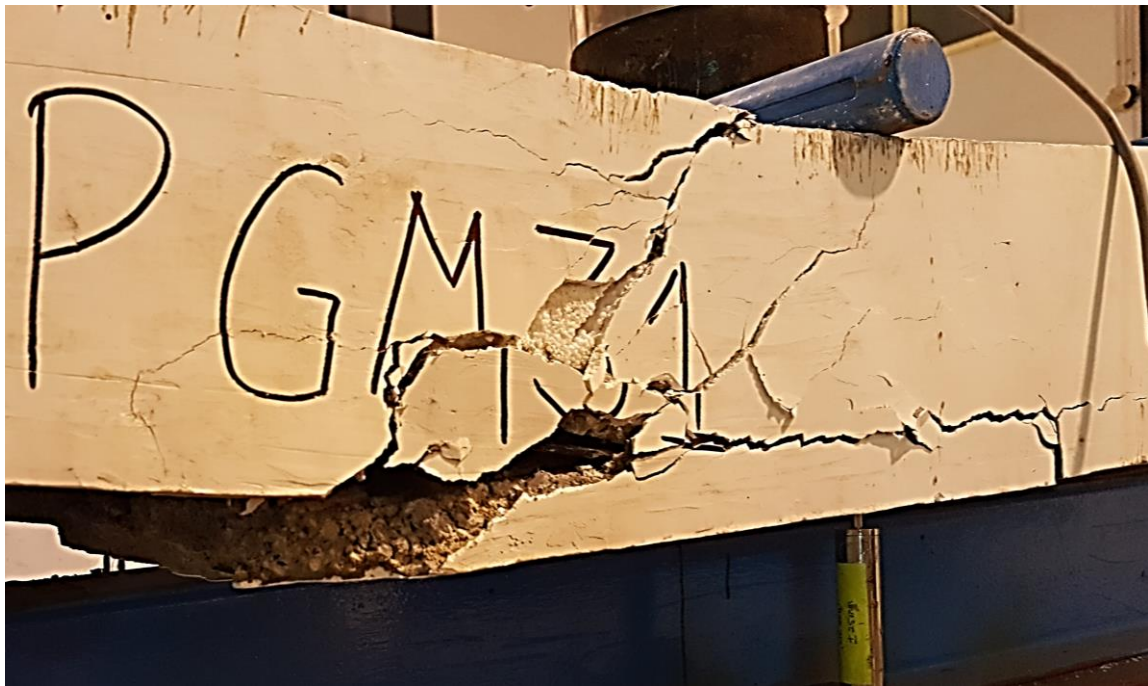
Figure 4. 12: Cracks propagation from the loading point towards the lower wythe through EPS
