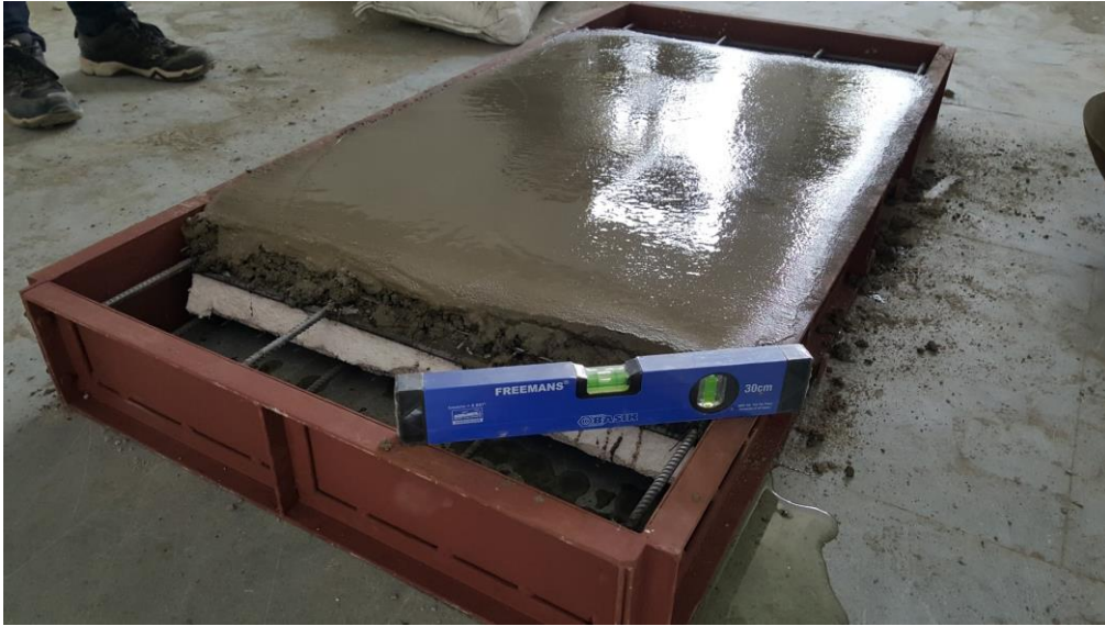
Figure 3. 25: Spirit level check during wythe casting.
