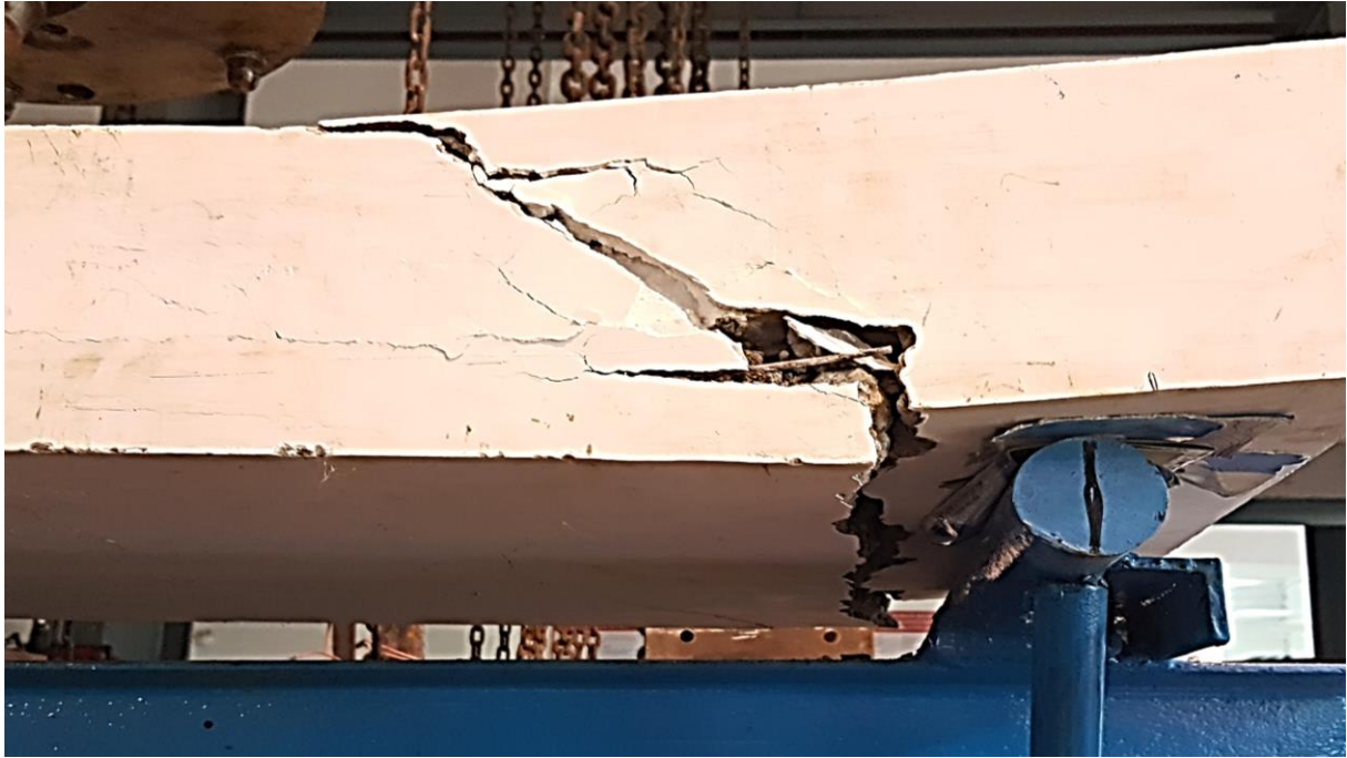
Figure 4. 11: Initial cracks appeared at the mid span and reaching the ultimate failure near the support
