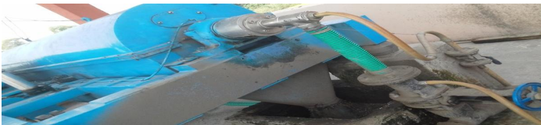
Fig 3.20 Polyelectrolyte mixing in centrifuge Unit
