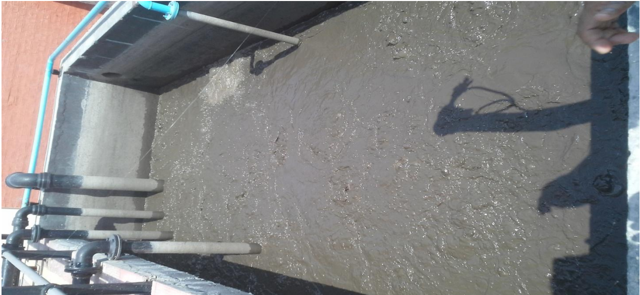
Fig 3.19 Sludge Sump
