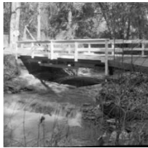
(a) Bridge image
