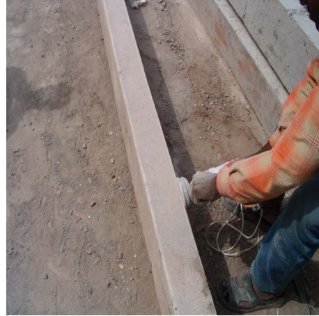
(b) Rounding of Edges of Beam-2
