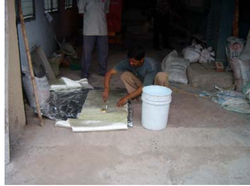
(a) Application of Epoxy Resin to Surface of Beam and GFRP Sheets
