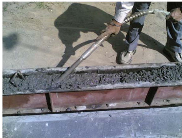
(e) Compaction of Concrete Using Needle Vibrator
