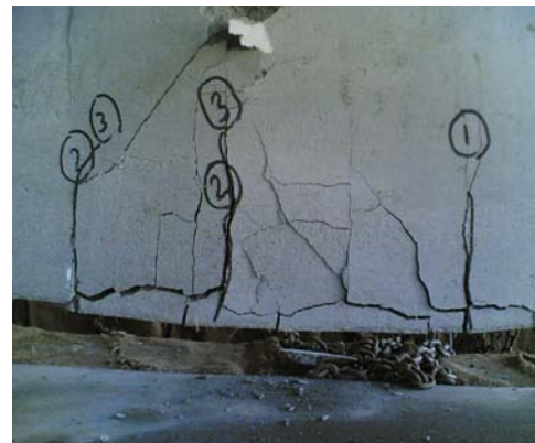
2B60(1)- Failure 1 (Spalling of Cover)
