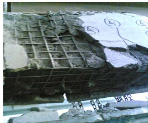
2B60(1)- Failure 3 (After removing cover)
