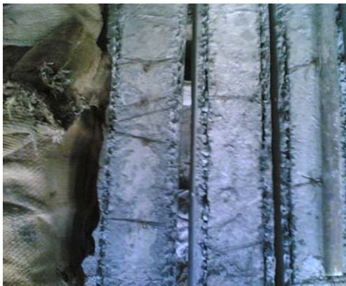
(c) Fixing of Wire Mesh - 1
