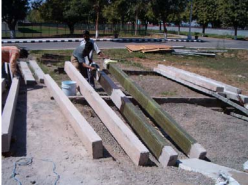
(a) Application of Epoxy Resin to Surface of Beam and GFRP Sheets
