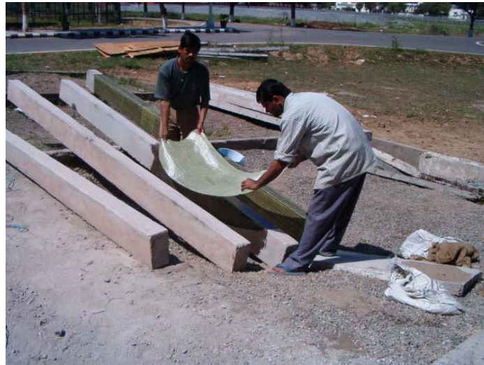
(b) Fixing GFRP sheets to the Beams
