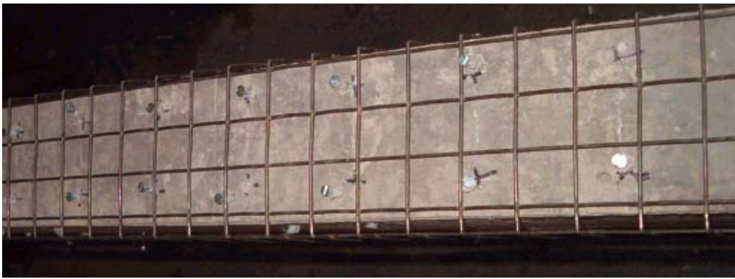
(c) Shear Connectors with cement Slurry as Bonding agent
