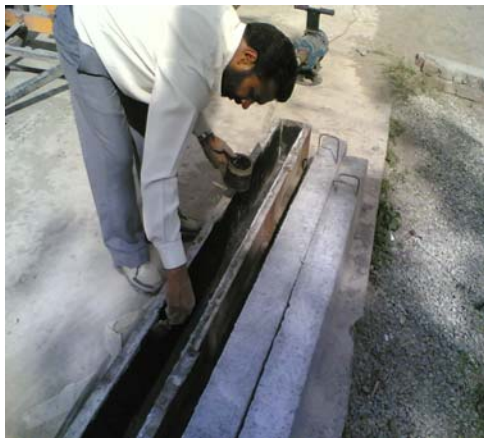
(c) Preparation of Moulds
