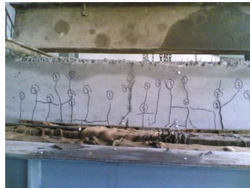
2U75 – at Failure 2
