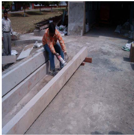
(c) Rounding of Edges of Beam-3
