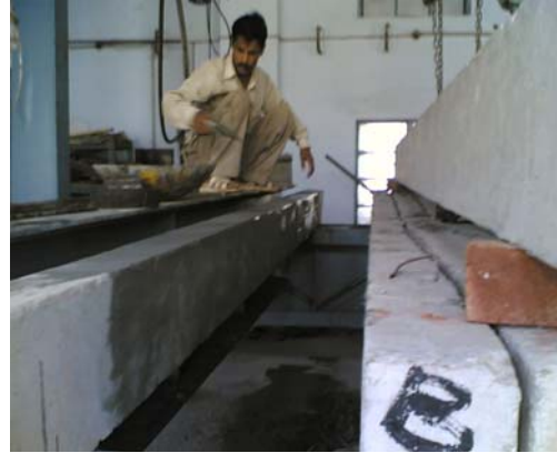
(b) Application of Cement Slurry
