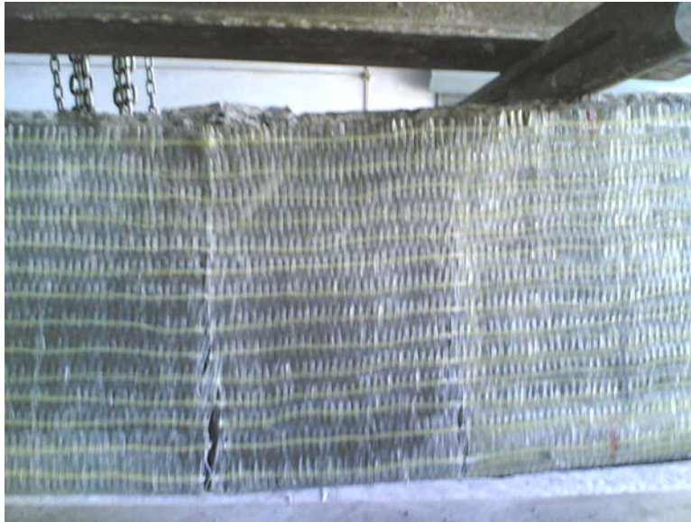
Plate 6.1 Failure of Beam Retrofitted with GFRP Jacket with Fibres at zero Degree to The Longitudinal Axis of Beam
