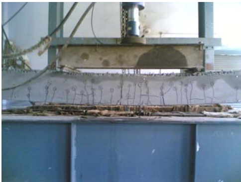
2U75 – at Failure 1
