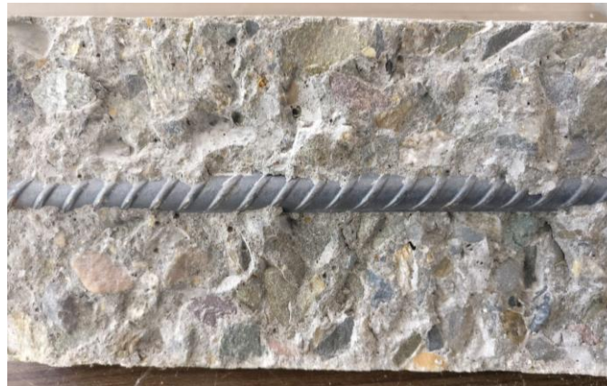
Figure 4.35 Rebar-concrete interface of NBAT specimen after 130 days of chloride exposure depicts no sign of corrosion initiation
