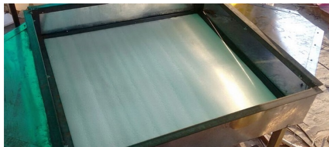
Fig 4.5: Insulating the rear of solar air heater.
