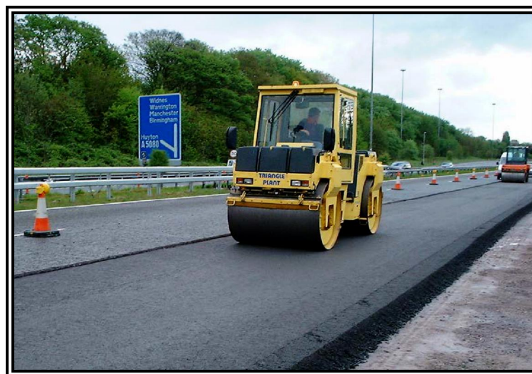
Fig. 2.6 Utilization of recycled asphalt in road construction
