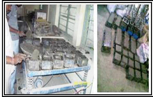
Fig. 2.3 Production of concrete blocks
