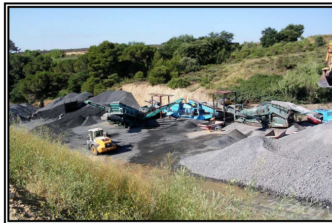
Fig. 2.7 Utilization of slag as road bed material
